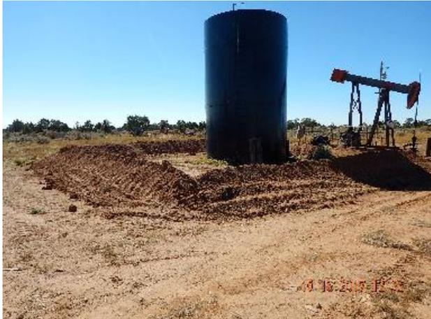
**Photo 5: Berms constructed around 400BBL tank..**
