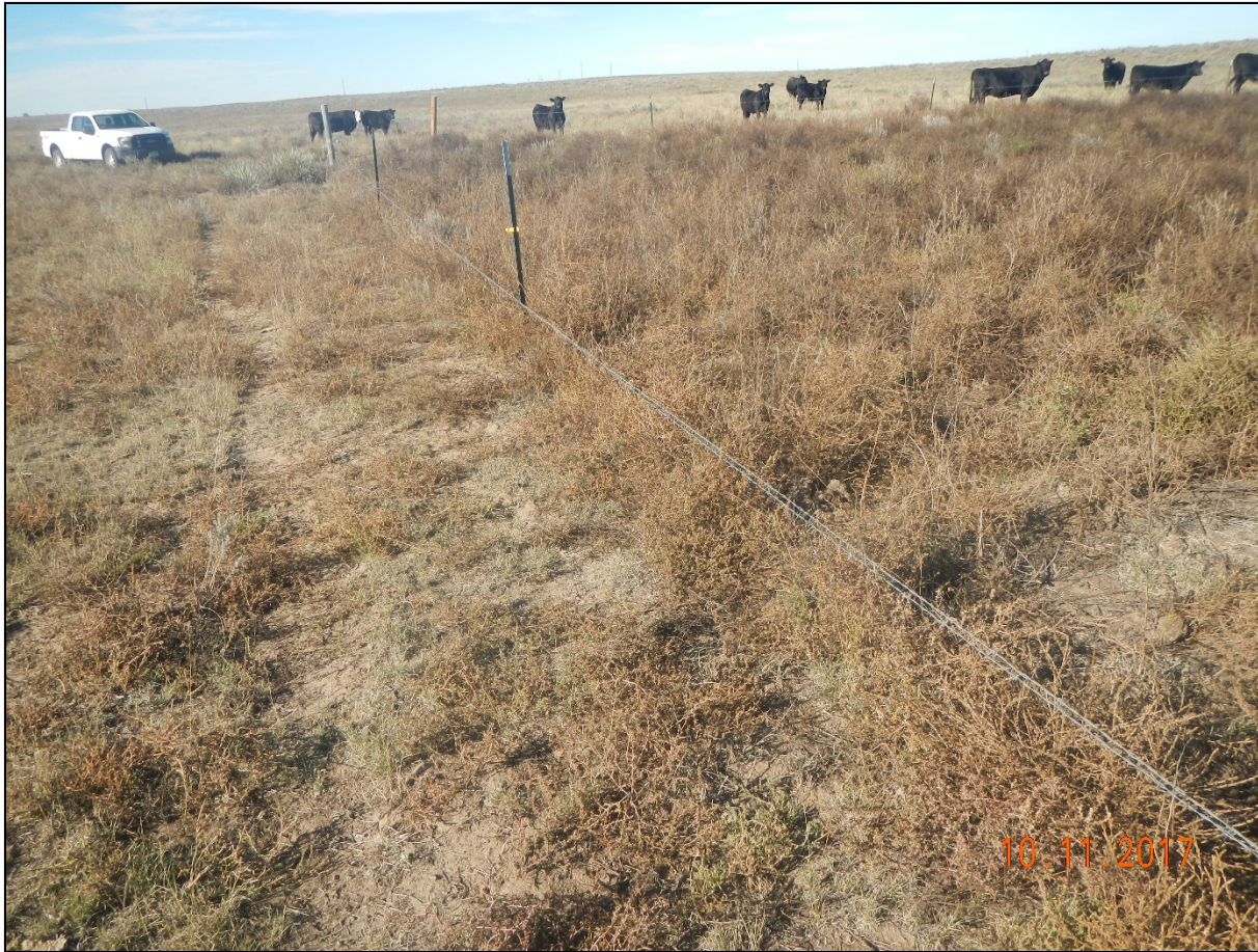
Photo 11. The fence around the location is not maintained. The barbed wire is only about 1 ft. off the ground and livestock can access the site.
