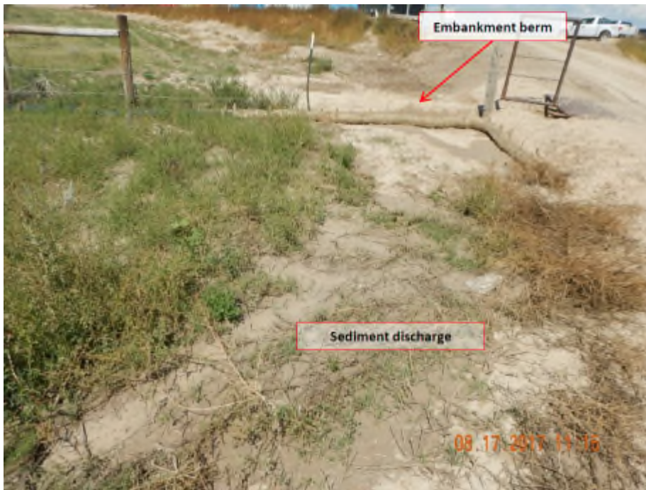
Photo 20. Photo taken east of the previously shown sediment trap in Photo 17. Photo illustrates sediment loss from stormwater overflowing from the sediment trap. Does not appear the wattles installed along the outer perimeter of the sediment trap are preventing sediment discharge. Wattles are intended to pool sheet flow (not filter sediment).
