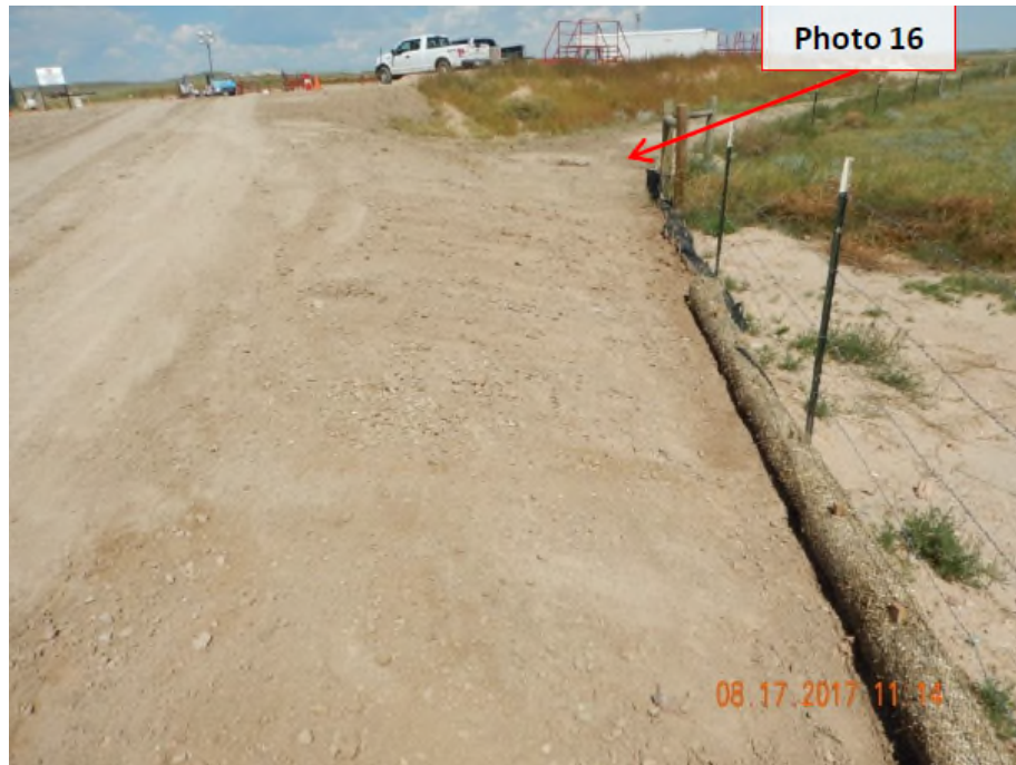
Photo 17. Photo taken from the west well pad, east entrance along the east side, facing Northwest. Appears the Operator has made repairs and re-installed wattles along the entrance.
