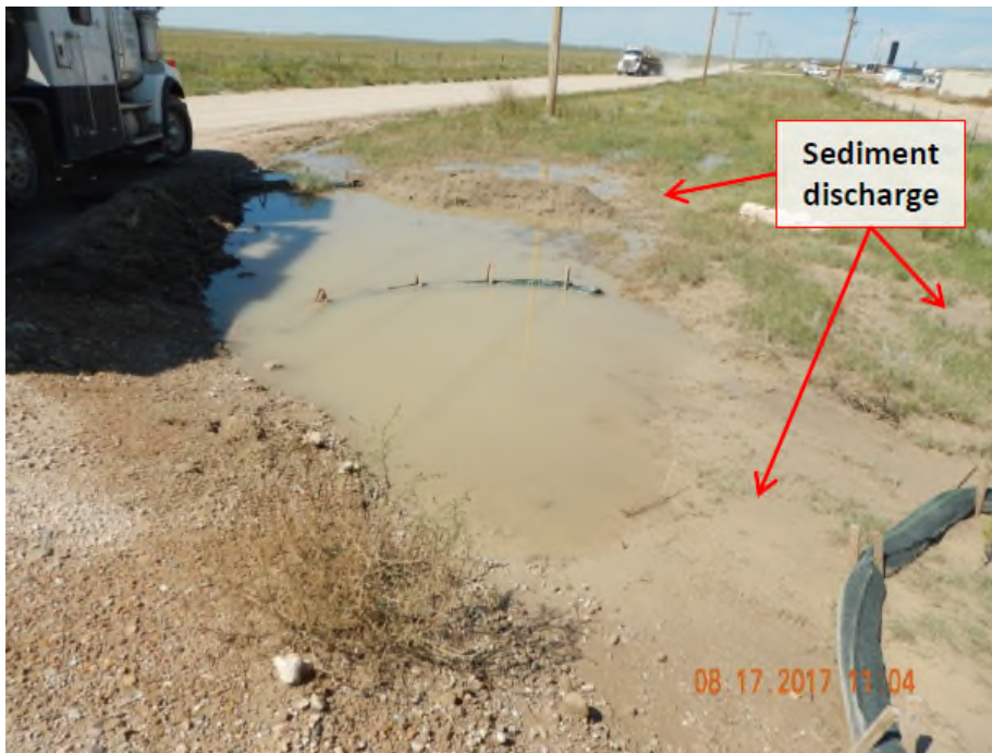
Photo 15. Photo taken from the previously shown sediment trap, facing Southwest. Does not appear the wattles are pooling stormwater runoff. Appears the volume of stormwater sheet flow is overtopping the wattle as shown in this photo. Sediment deposition is observed between the wattles and outside of the wattles as shown in this photo.
