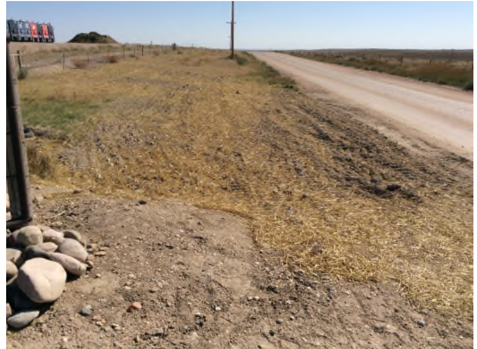
Photo NBL13. Ponding in this area was due mainly to run-on from the lease road. To address this issue, the elevation of the area was raised to remove the low spot where water would pool. The wattles were removed, and the area was seeded and crimped
