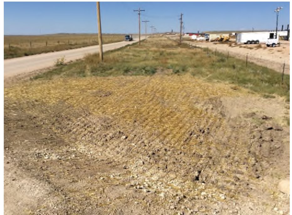
Photo NBL15. Ponding in this area was due mainly to run-on from the lease road. To address this issue, the elevation of this area was raised to remove the low spot where water would pool. The wattles were removed, and the area was seeded and crimped
