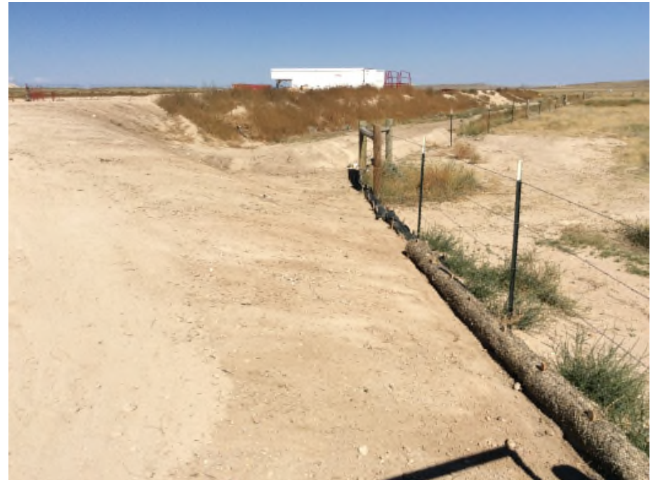
Photo NBL17. The rock socks and wattles were maintained
