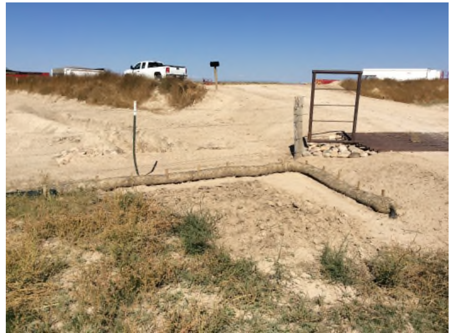
Photo NBL20. The straw wattle was maintained and rock was installed at cattle guard. Sediment was also recovered.
