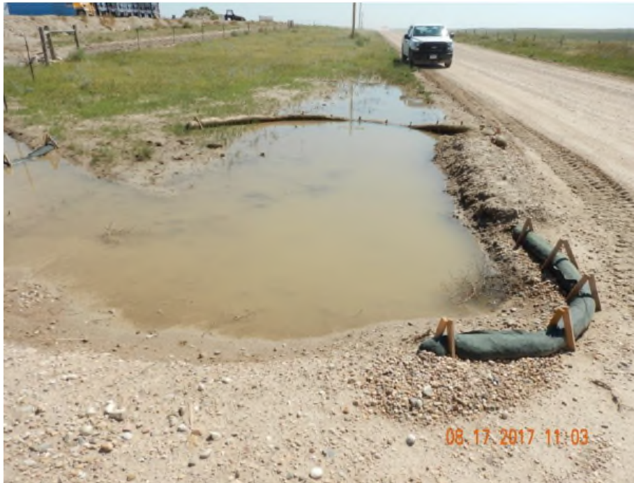
Photo 13. Photo taken from the previously mentioned shallow depression area, facing East. Does not appear the depression area with the wattles are pooling stormwater runoff. Appears the volume of stormwater sheet flow, likely sediment laden flow, is overtopping the wattle as shown in this photo.
