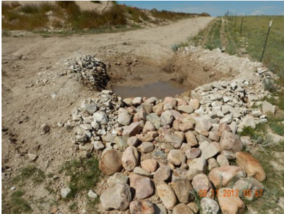
Photo 9. Photo taken from the northeast east well pad, facing West. Appears the Operator has enlarged the sediment trap size with a stabilized outlet area. Embankment material and embankment construction does not appear to be sufficient compacted, as it appears unconsolidated material could be contributing to sediment loss. Refer to Photo 10 for a picture taken of the sediment trap from the July 11, 2017 inspection.
