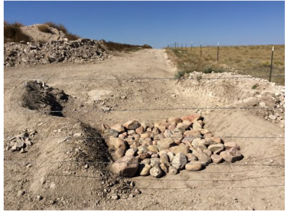
Photo NBL9. The sediment trap was enlarged and berms around the trap were compacted.
