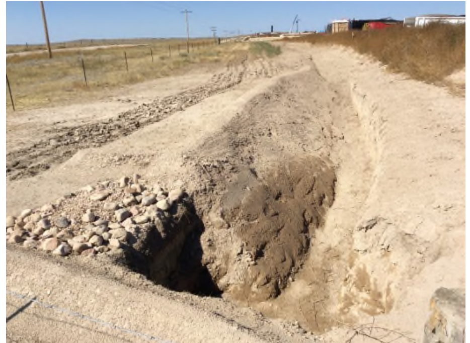
Photo NBL18. The sediment trap was enlarged and extended, and the embankment was raised and re-compacted.
