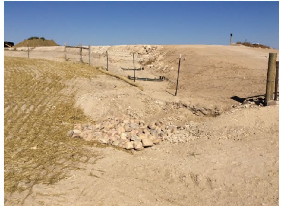
Photo NBL2. A straw wattle was installed to help direct runoff from the upgradient sediment trap into the secondary sediment trap. The area between the traps was cut lower as well to contain runoff between the traps.
