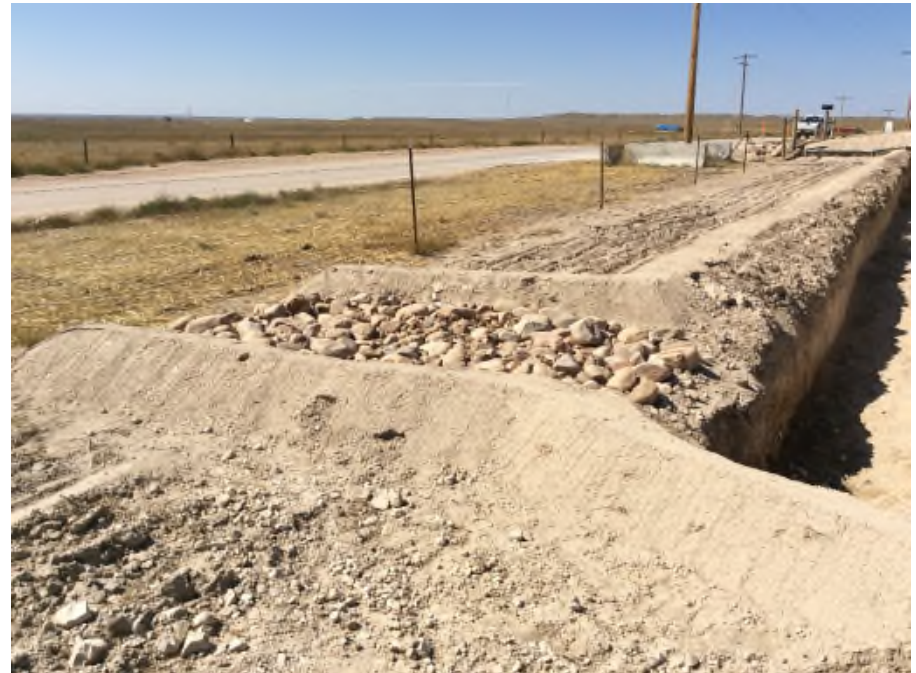
Photo NBL10. The outfall for this trap was extended and the trap was enlarged.
