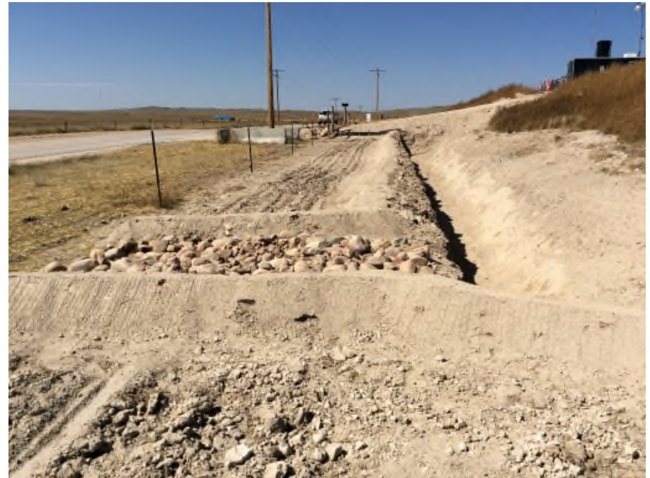
Photo NBL9. The sediment trap now spans the front of pad and is approximately 3.5' deep across the face of pad. The berms were re-compacted and extended North
