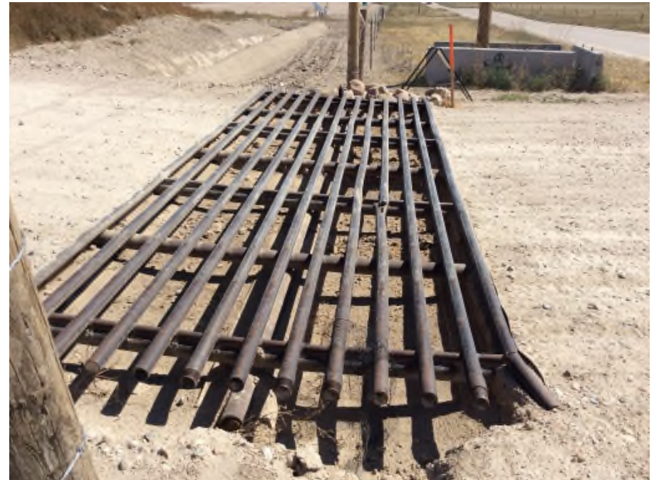
Photo NBL7. The cattle guard was cleaned out
