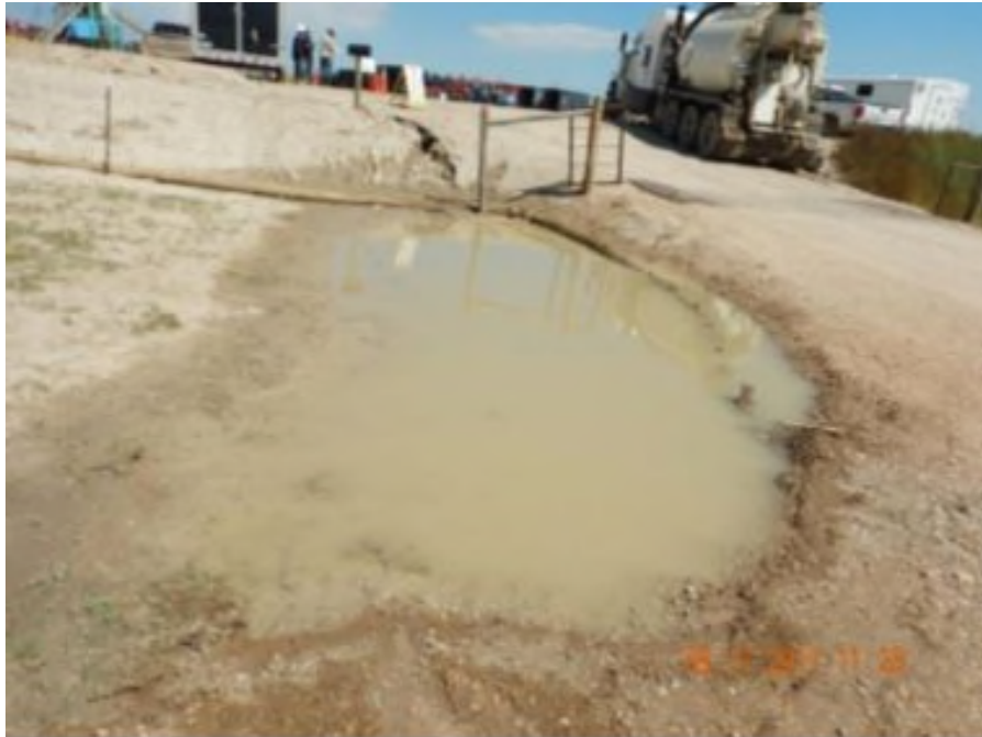
Photo 6. Photo taken from the entrance of the Tombstone pad, along the west side, facing North. Sediment discharge observed, as the wattle BMP does not appear to be sufficient.
