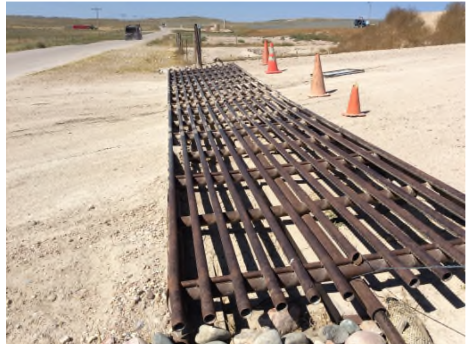
Photo NBL11. The cattle guard was cleaned out and rock was installed on the sides of the cattle guard
