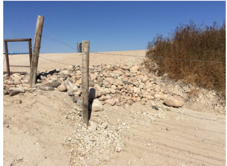
Photo NBL3. Rip rap was installed to prevent gully erosion
