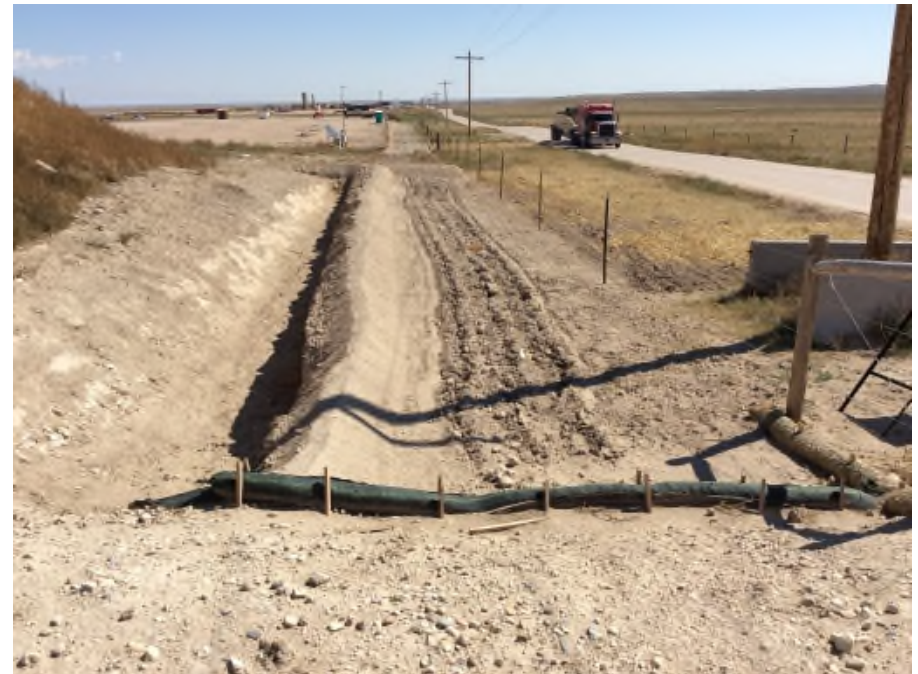
Photo NBL8. This sediment trap was combined with the sediment trap in the SE corner. The ripping was maintained
