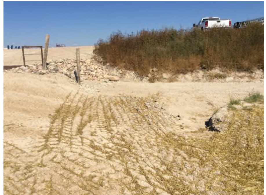
Photo NBL2. Rip rap was installed on the side of the lease road to prevent gully erosion. The sediment trap was removed to bring the BMPs inside the disturbance footprint; however, other sediment traps that were enlarged account for the volume lost by removing this sediment trap. The ditch shown will carry runoff to the sediment trap in the SE corner
