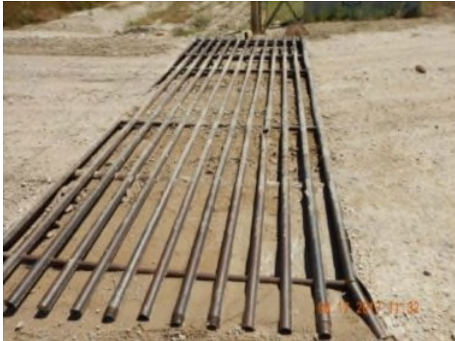
Photo 7. Photo taken from the cattle guard of the Holliday east entrance, facing East. Cattle guard in need of maintenance.
