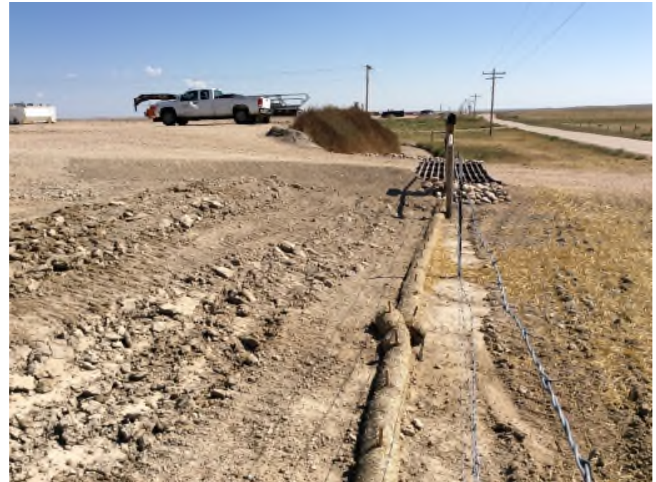
Photo NBL5. The berm was extended to direct runoff to the cattle guard, straw wattles were maintained, ripping was installed, and the slope was re-graded to approximately 2:1
