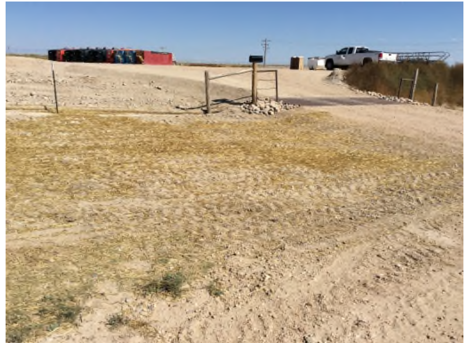
Photo NBL6. This pooling was, in part, the result of run-on from the lease road. This area was seeded and crimped, and the depression was filled to prevent pooling
