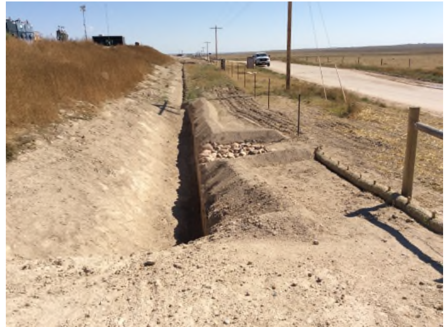
Photo NBL12. The trap outfall was moved east to allow proper drainage. The trap was enlarged (depth and length) and the area outside the disturbance seeded and crimped
