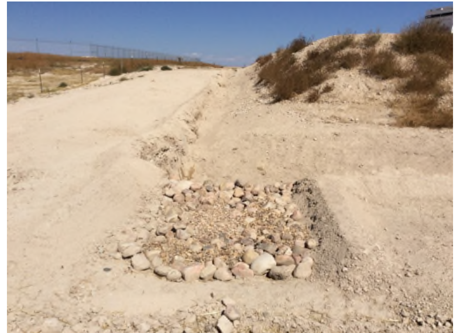
Photo NBL13. The trap was enlarged, the berms were re-compacted, the rock sock was removed, and the area just outside the outfall was seeded and crimped after sediment was recovered
