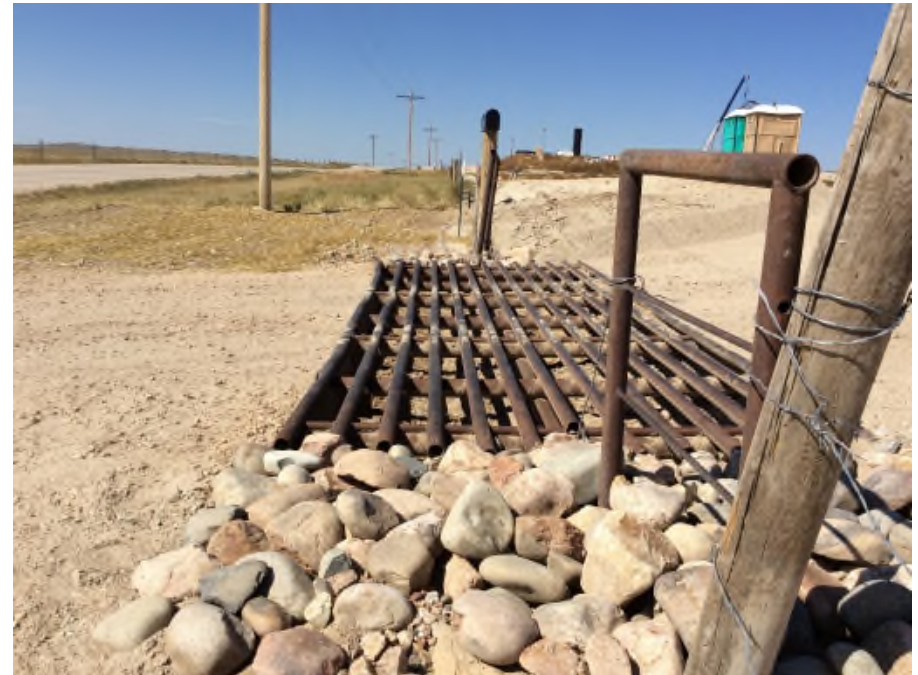
Photo NBL4. The cattle guard was cleaned out and rock was installed on the edges of the cattle guard.
