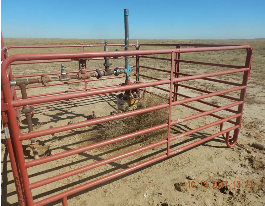
Photo 1: Wellhead, looking NE, no wellhead sign or emergency contact number
