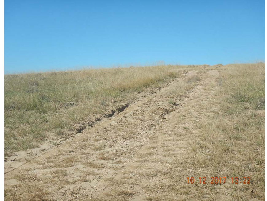
Photo 2: Stormwater erosion along access road
