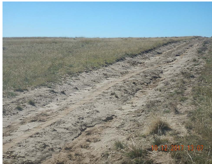
Photo 2: Stormwater erosion along access road
