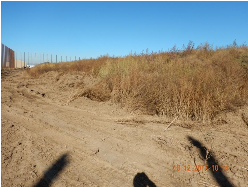
Photo 1. Photo taken from the southeastern location, facing West. Photo illustrates the southern topsoil stockpile is not being protected from weed establishment per Rule 1002.c. Topsoil stockpile has significant weed cover- Russian thistle and Kochia.
