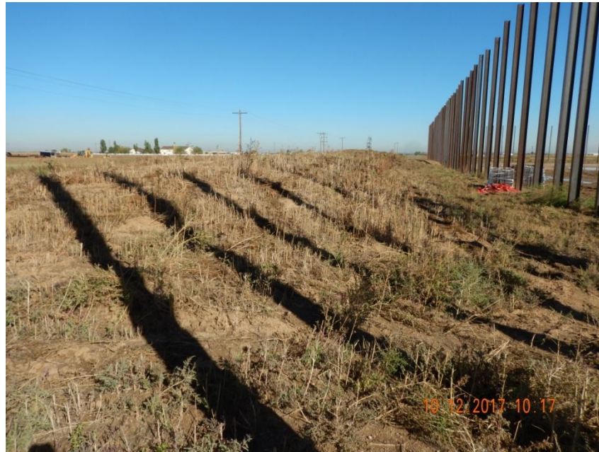
Photo 3. Photo taken from the southwestern location, facing North. Photo illustrates the western topsoil stockpile is not being protected from weed establishment per Rule 1002.c. Topsoil stockpile has significant weed cover- Russian thistle and Kochia.
