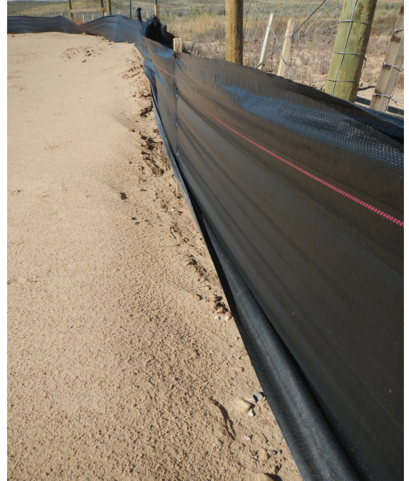
Portions of Fence showing poor installation
