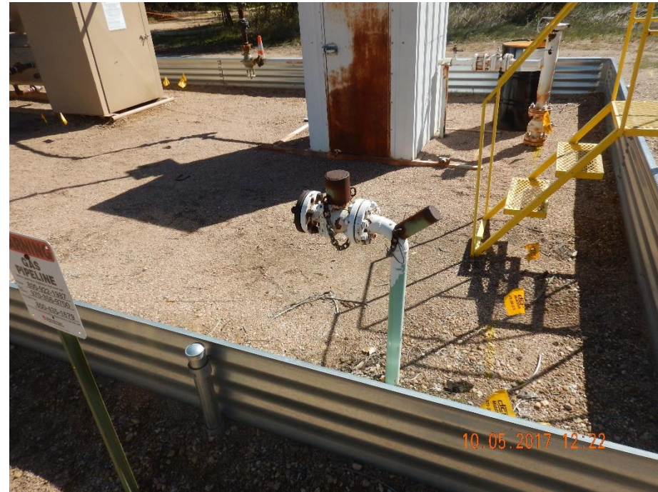
Photo 2: Photo taken from the battery location. Photo shows riser requiring removal.
