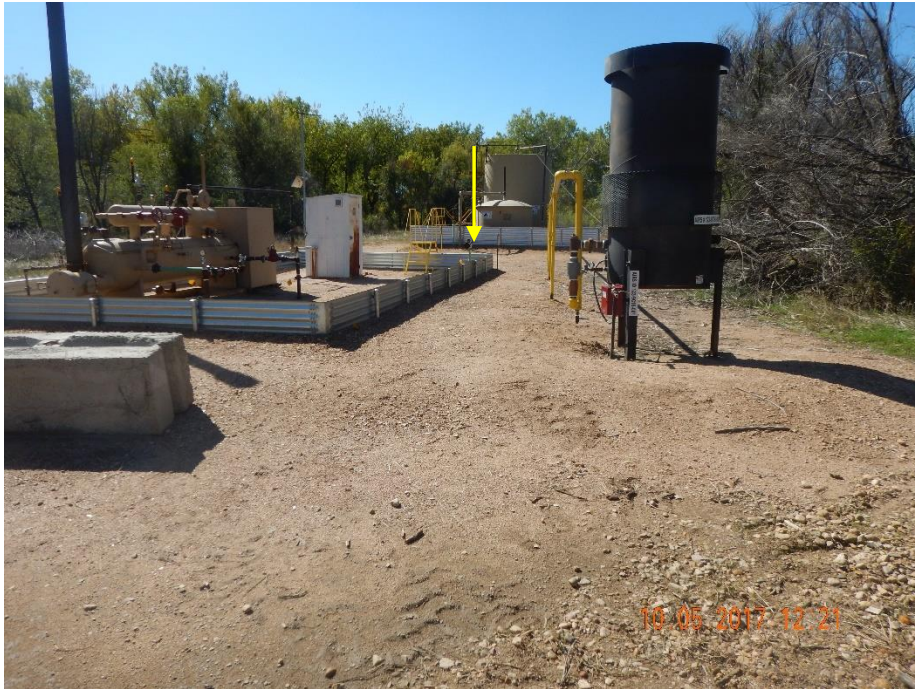
Photo 1: Photo taken from the east end of the battery location. Arrow indicates location of riser requiring removal.
