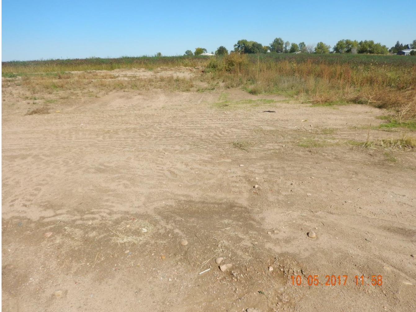
Photo 1: Photo taken from the former well, facing north. Photo shows riser identified in the previous inspection has been removed per the corrective action. Location still requiring reclamation including re-contouring/re-grading and revegetation.
