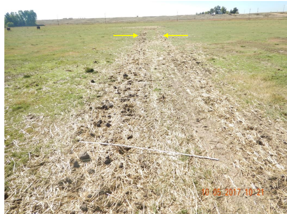
Photo 4: Photo taken north of the well location, facing south. Photo shows well and access road appears to have been reseeded and stabilized via crimped straw. Photo also shows areas of the access road where the ruts remain visible, this suggests the required compaction alleviation may not have been performed per reclamation rules. Reclamation will not pass until the required compaction alleviation of the access road and well have been performed.
