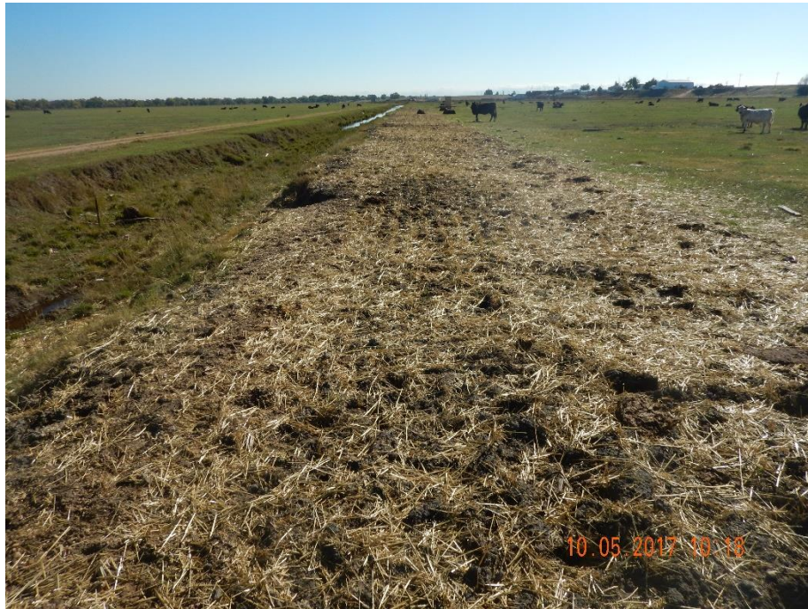
Photo 3: Photo taken from the east end of the former battery location, facing west. Photo shows access road appears to have been re-seeded and stabilized via crimped straw.
