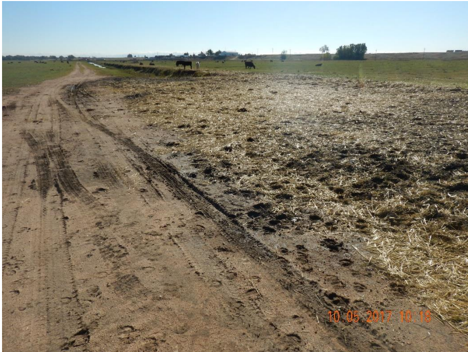
Photo 1: Photo taken from the northwest end of the former battery facility, facing southeast. Photo shows areas appear to have been re-seeded and stabilized via crimped straw.
