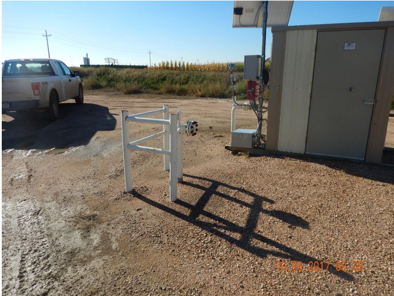
Photo 1: Photo taken from the western portion of the battery facility, facing south. Photo shows pipe riser equipment that appears to be abandoned. Riser needs to be removed in accordance to COGCC rule 1004.a
