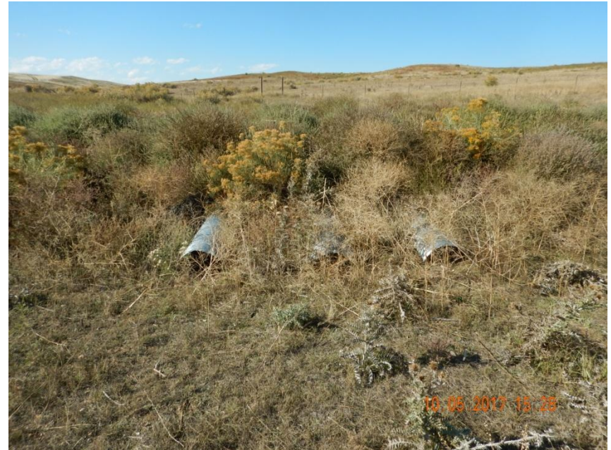
Photo 4. Photo taken along the portion of access road that intersects with an intermittent stream, facing North. Culverts have not been removed.
