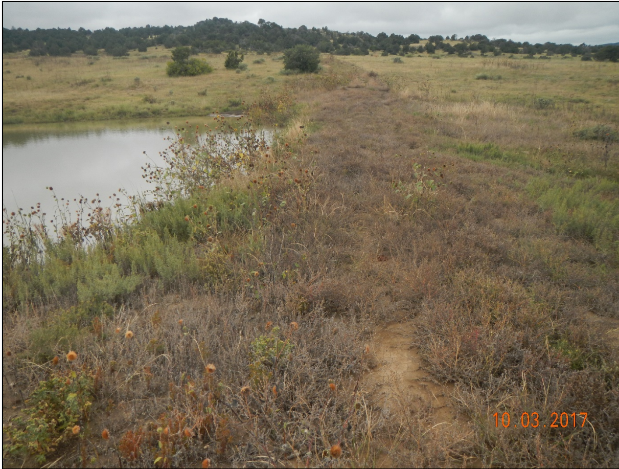
Photo 6. Facing southwest along the access road. There is stormwater held back by the road on the eastern side. There is a potential for stormwater to flow across the road causing erosion however there was minimal signs of this occurrence.
