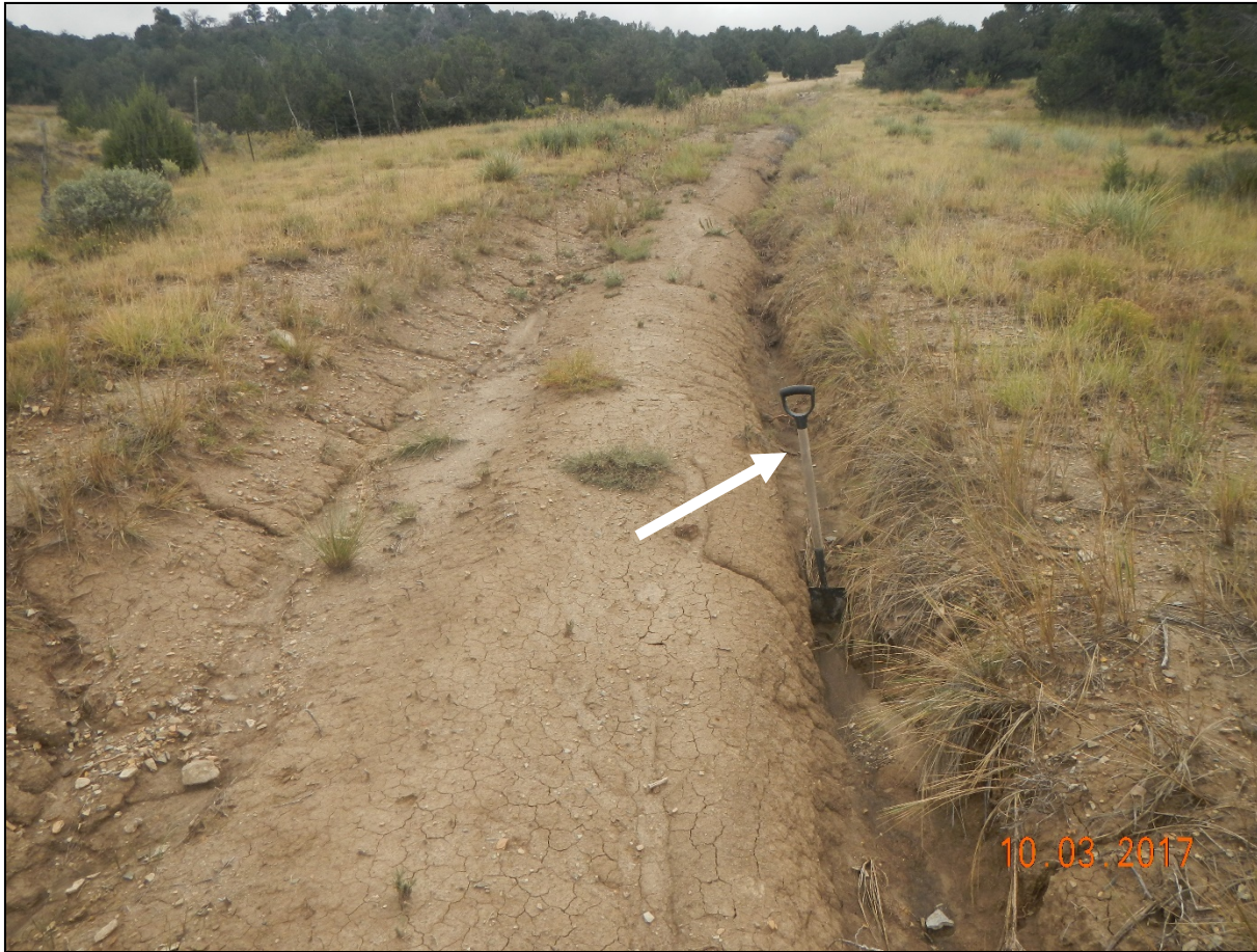
Photo 9. There is erosion occurring down the slope of the road. The arrow points to a 3.5 ft. shovel in the erosion channel which indicates depth.
