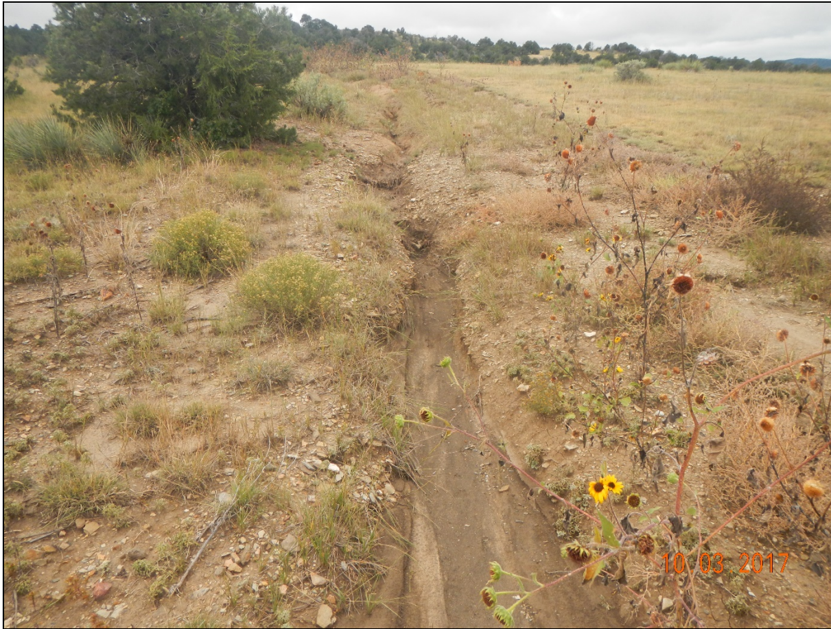
Photo 7. Facing southwest along the access road where it gradually ascends. There is erosion occurring from this point at the bottom of the slope all the way to the top near the location. Approximately 1500 ft.
