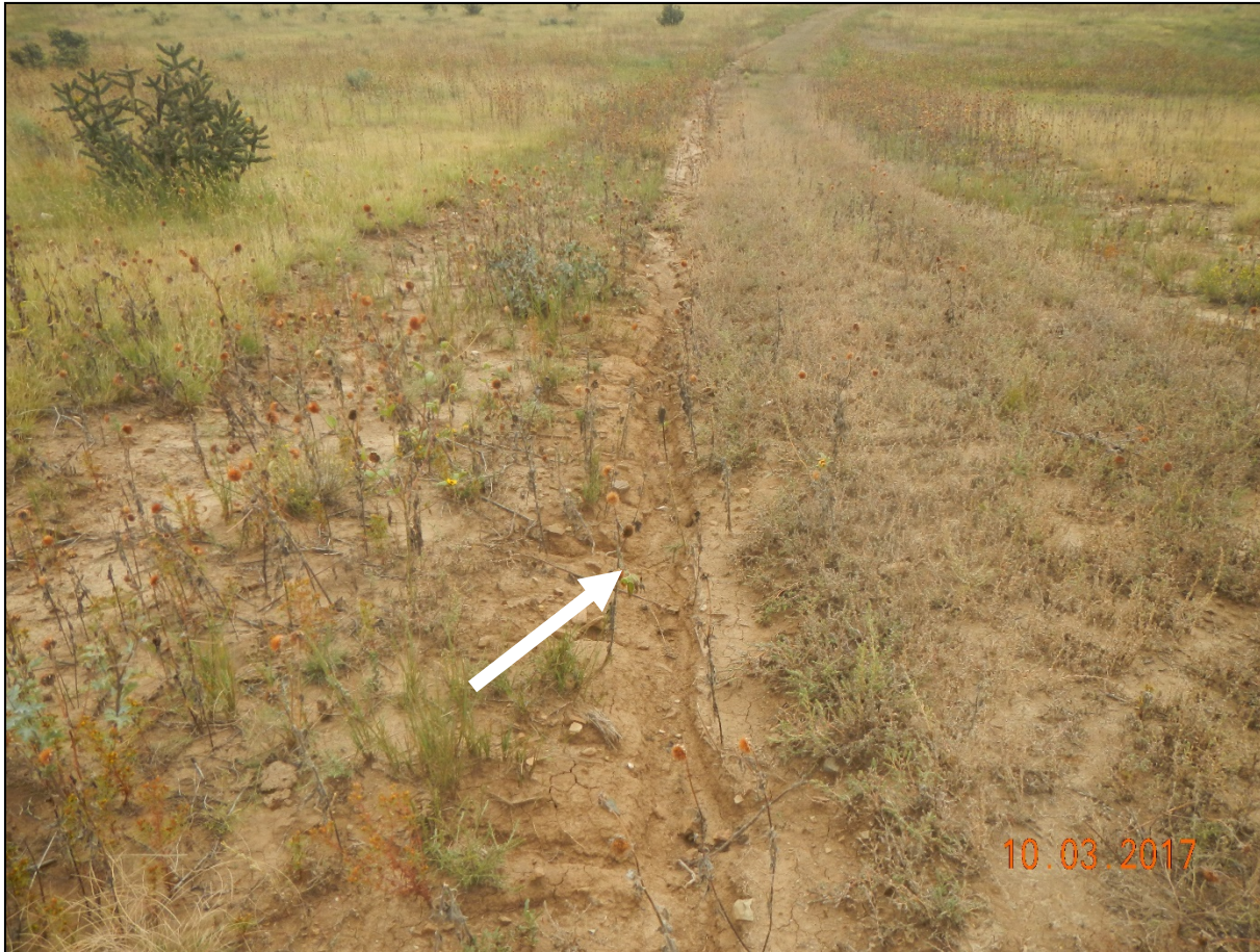
Photo 5. There are signs of stormwater erosion occurring along the road.
