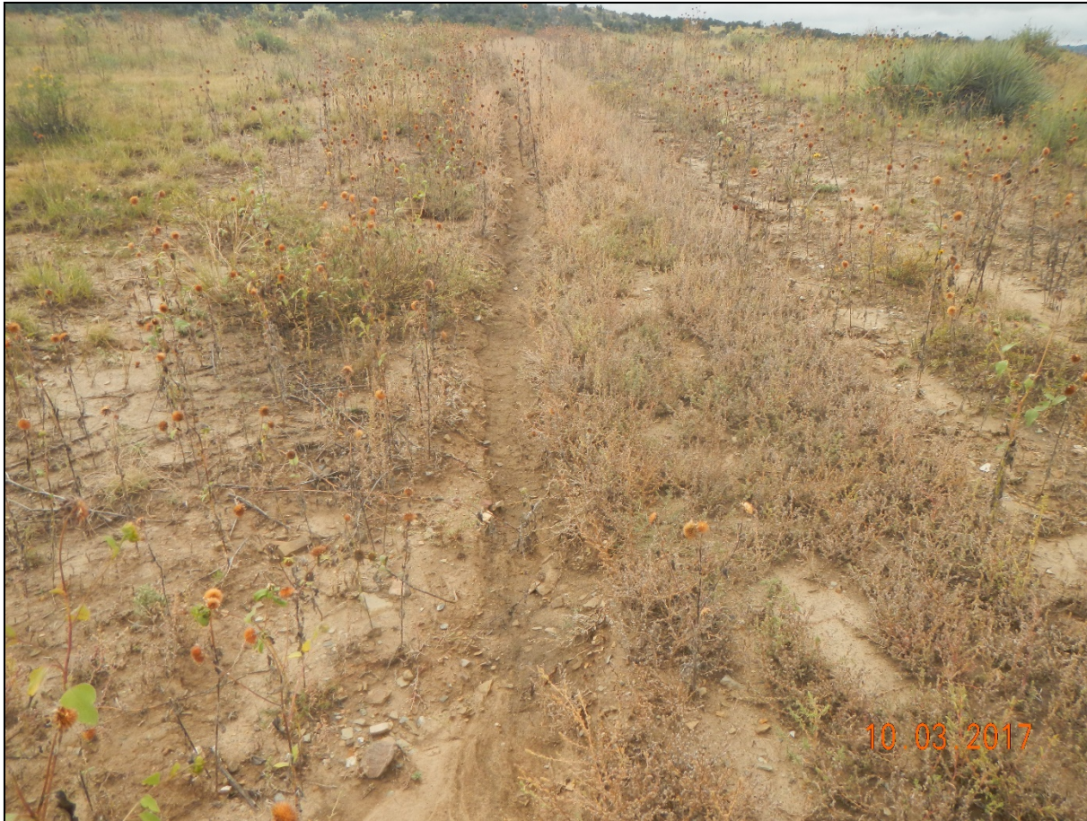
Photo 7. Facing southwest along the access road where it gradually ascends. There is erosion occurring down the slope of the road.
