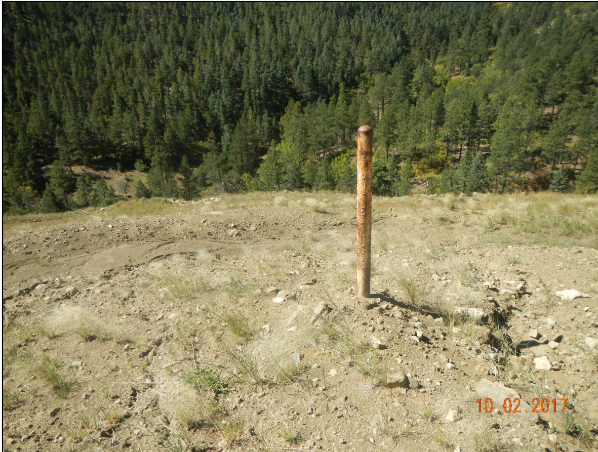
Photo 17. There is erosion occurring near the well marker.
