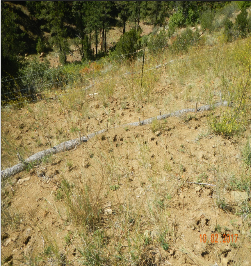
Photo 5. This area along the access road has less vegetation and erosion issues beginning to occur. The straw wattles have filled in with sediment.
