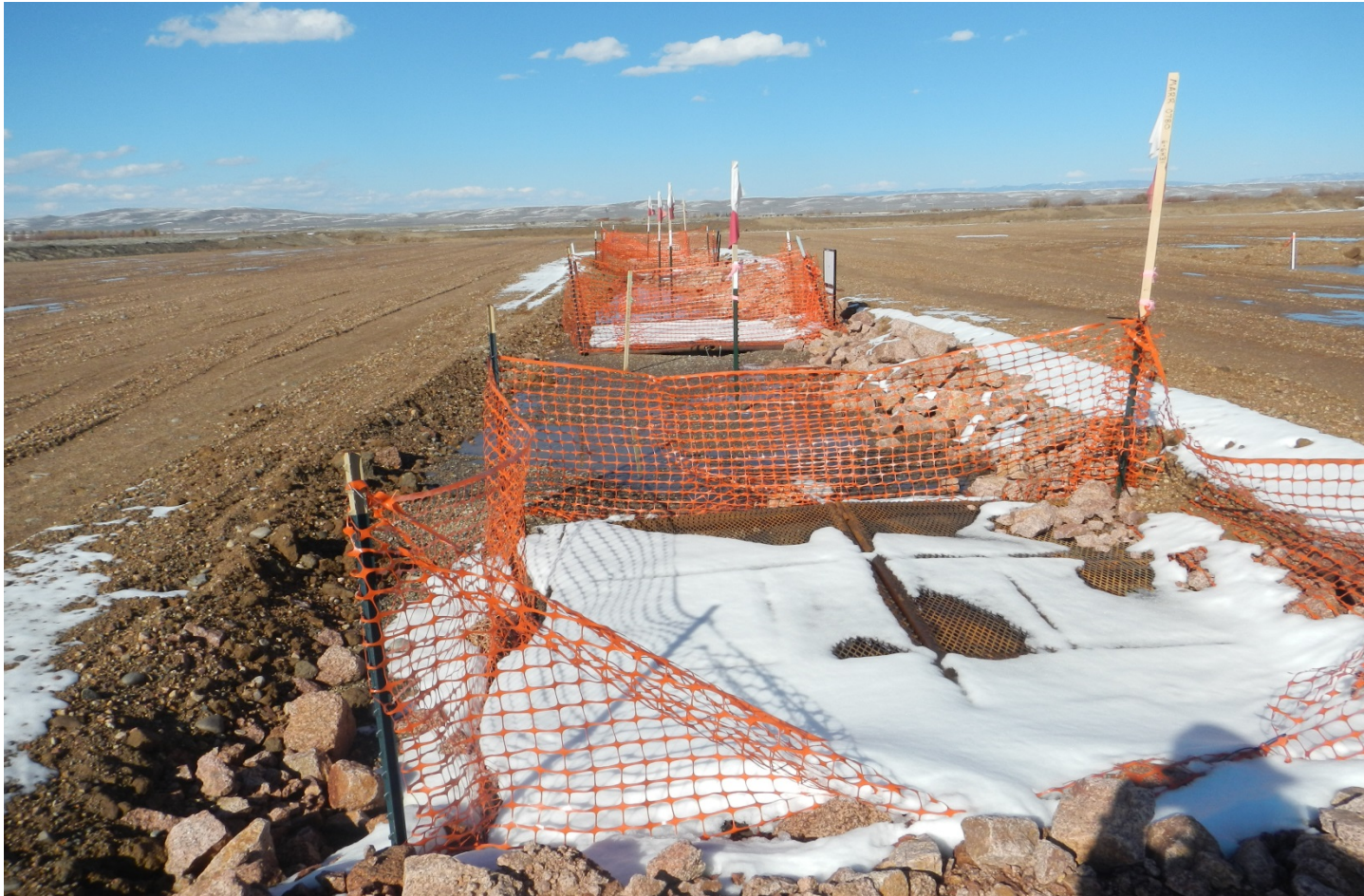
Photo#6: Conductors Set with Cellar Covers Installed.
