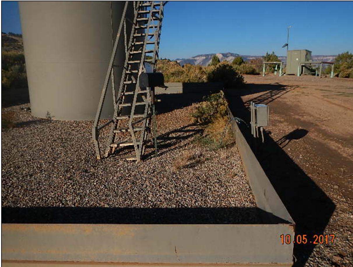
Photo 1. Vegetation in tank containment. Noted on two previous inspections for former operator.
