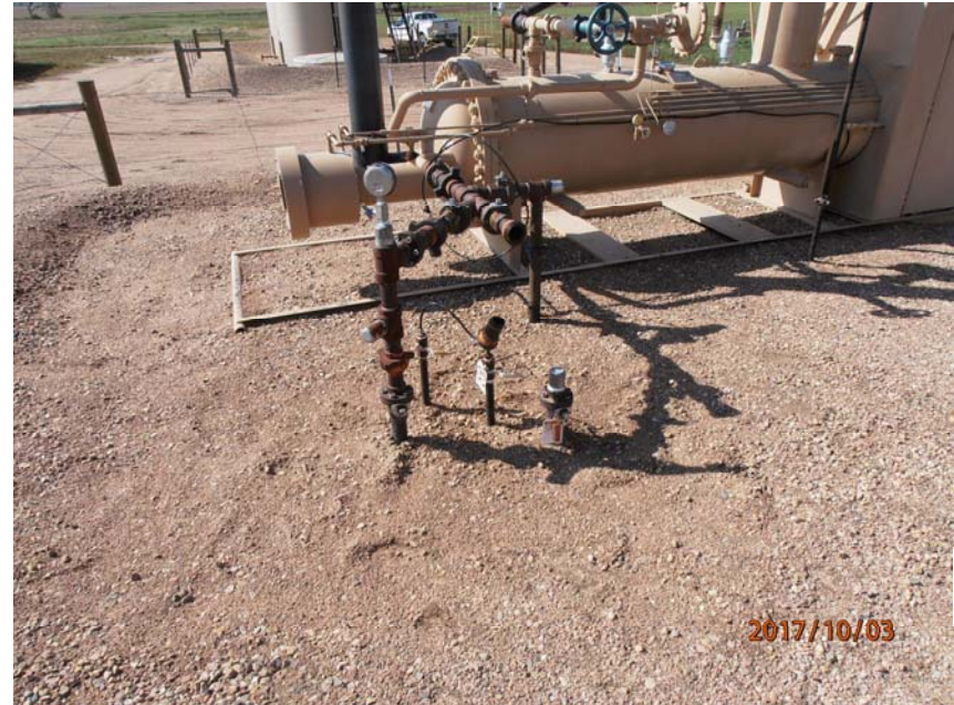
Photo 6: Flowline of Meyring 13-27 disconnected at separator.
