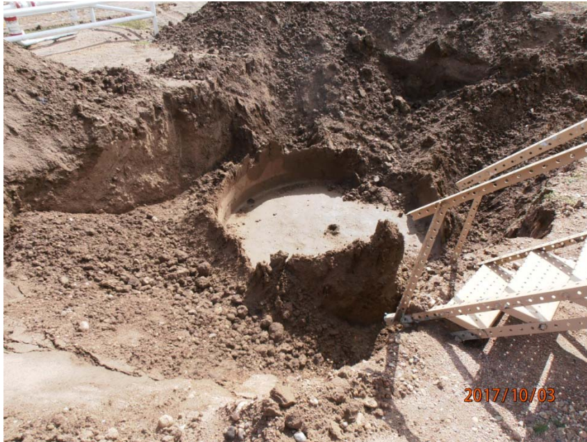
Photo 3: Partially buried produced water vessel excavation.
