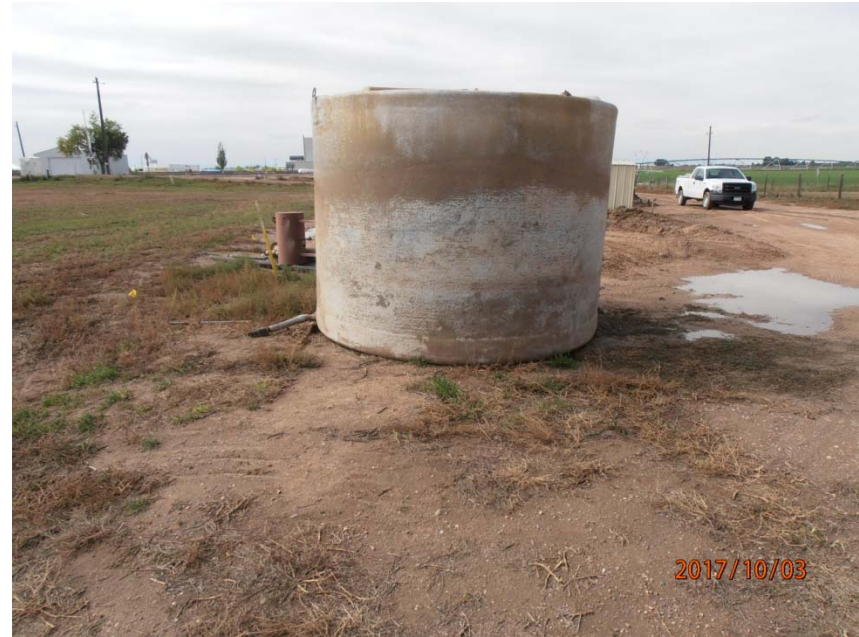
Photo 4: Fiberglass produced water vessel removed from excavation.
