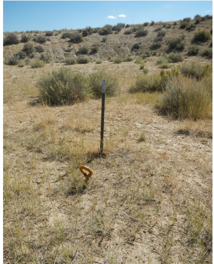
Photo#5: Guy Line Anchors on Location.
