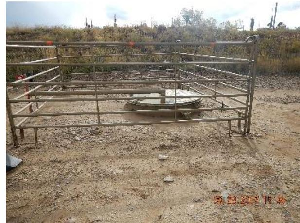
**Photo 6: Partially buried 21 BBL steel tank with no containment berms.**
