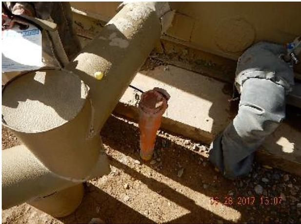
**Photo 5: Painted, capped, and tagged unused riser at separator.**
