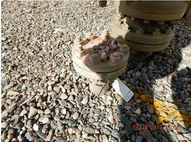
**Photo 3: Painted, capped, and tagged unused riser between separator and compressor building.**
