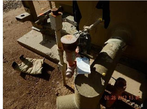
**Photo 4: Painted, capped, and tagged unused riser at separator.**
