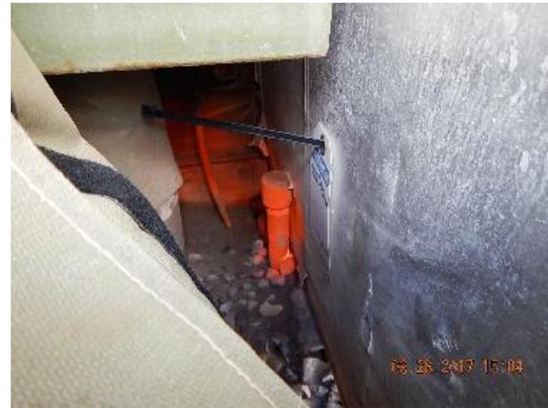
Photo 2: Painted, capped, and tagged unused riser. 1" riser in water box.
