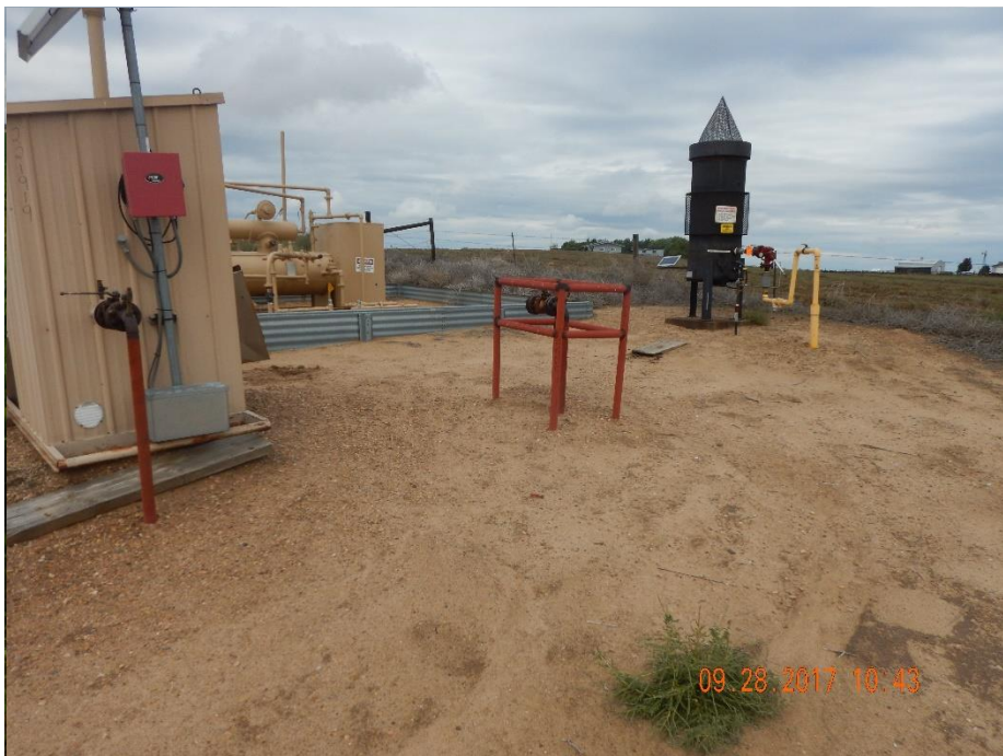
Photo 1: Photo taken from the west end of the battery location, facing northwest. Inspection doc. #682502147 and #675103862 required operator to remove riser at the battery in accordance to 1004.a reclamation requirements. Photo shows riser has not been removed.
