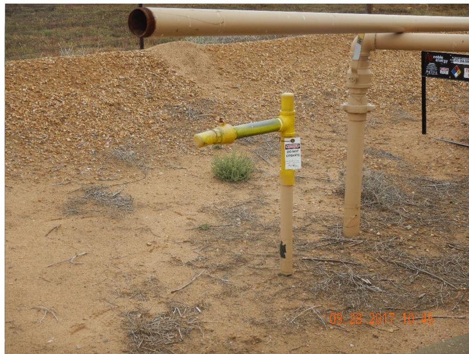
Photo 2: Photo taken from the east end of the battery location within the tank berm. Photo shows pipe riser that has been tagged and painted per the 2017 Flowline NTO, but has not been removed per the NTO required dates. This riser will need to be removed per the NTO and per 1004.a reclamation rules.
