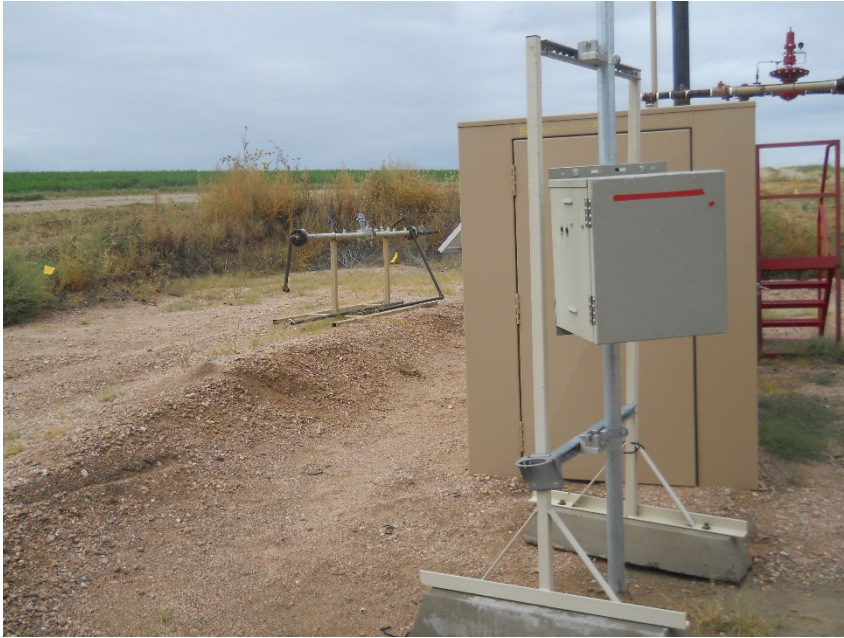
Unused piping and automation equipment south and east of south separator
