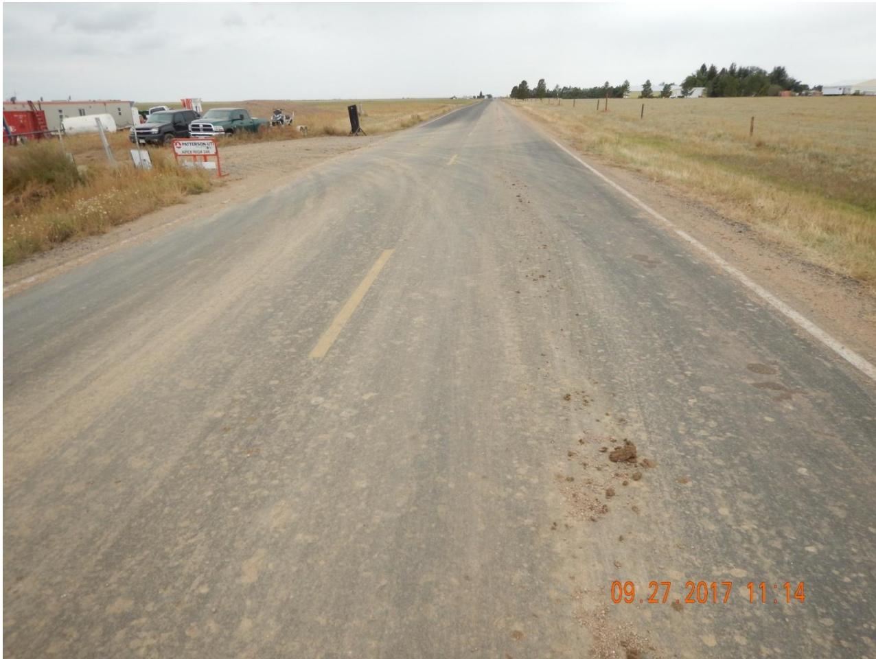
Photo 1. Photo taken from the entrance of location on CR 136, facing West. Tracking pad not adequately maintained to prevent tracking of material offsite.
