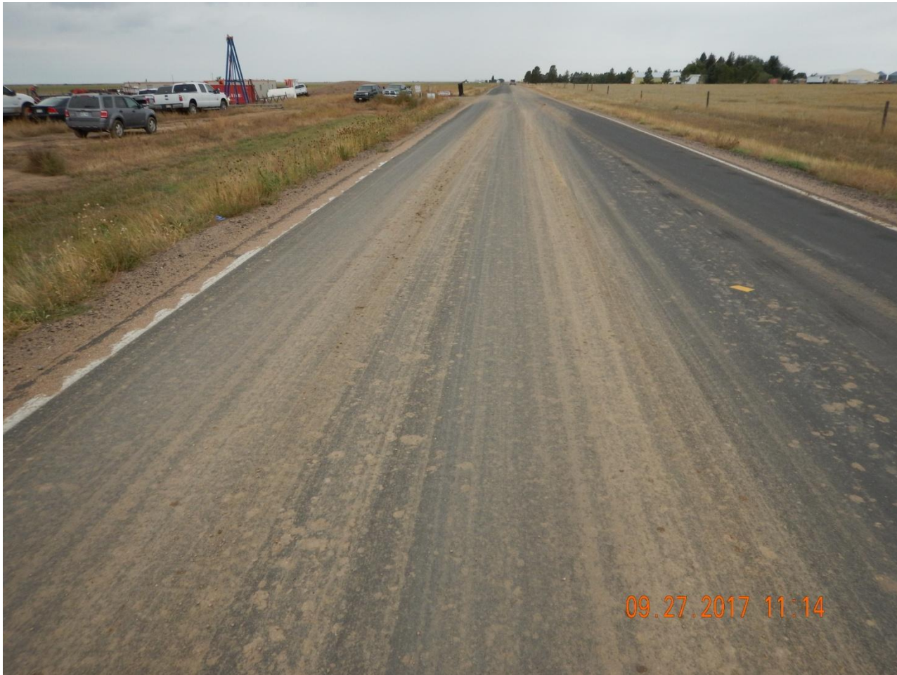
Photo 2. Photo taken from CR 136 east of entrance, facing West. Tracking pad not adequately maintained to prevent tracking of material offsite.
