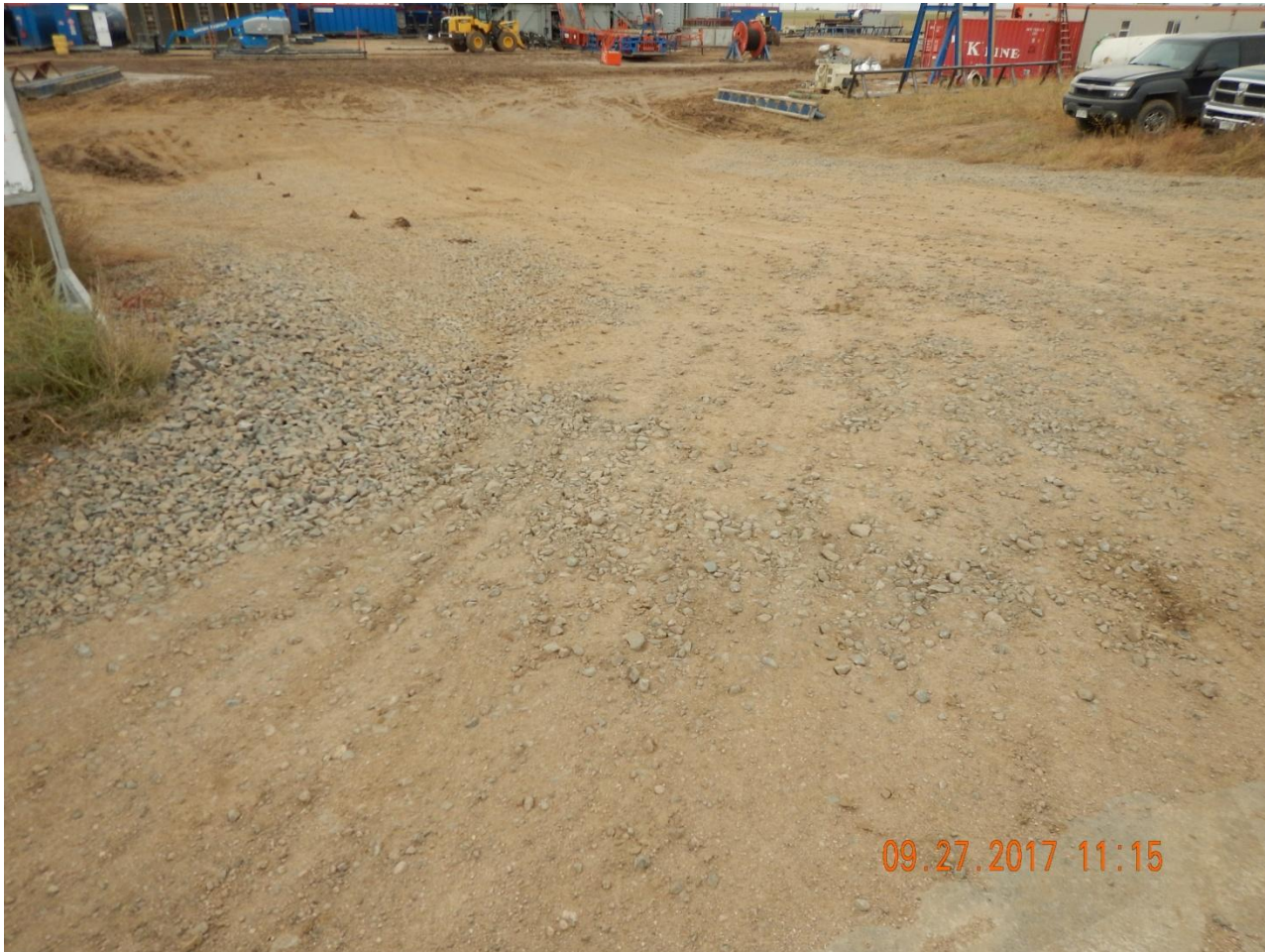
Photo 4. Photo taken from the entrance of location, facing South. Photo illustrates tracking pad not adequately maintained to prevent tracking of material offsite.
