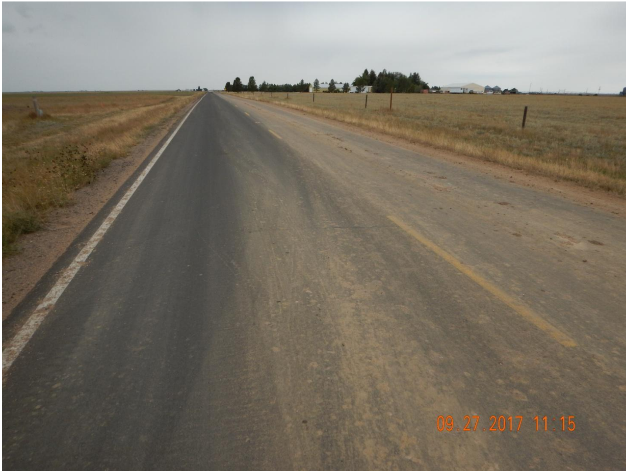
Photo 3. Photo taken from CR 136 west of entrance, facing West. Tracking pad not adequately maintained to prevent tracking of material offsite.
