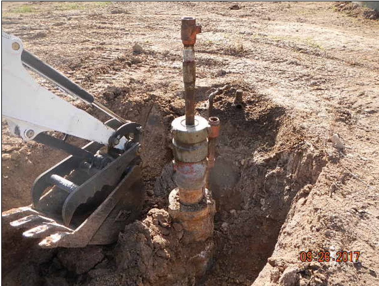
Photo 1. Well has been plugged, but had not been cut off and buried at time of inspection.
