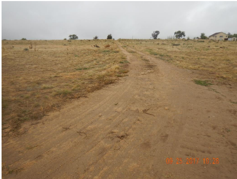
Photo 2: Photo taken from the northwest end of the location, facing west. Photo shows access road has not been reclaimed per COGCC 1000 series reclamation rules and requirements. Corrective actions have not been addressed.
