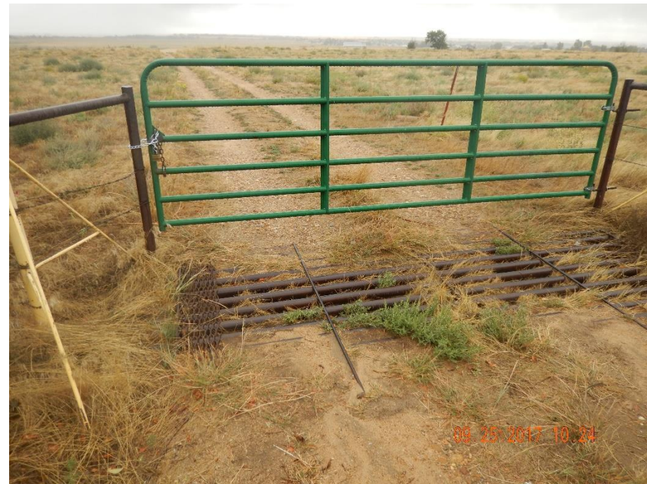
Photo 3: Photo taken from the access road entrance, west of the location. Photo cattle guard and gate remains; access road has not been reclaimed per COGCC 1000 series reclamation rules and requirements. Corrective actions have not been addressed.
