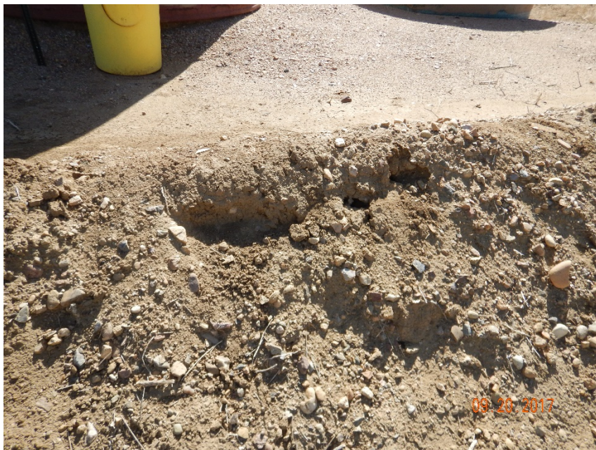
Photo #7 – Eroded earthen berm.
