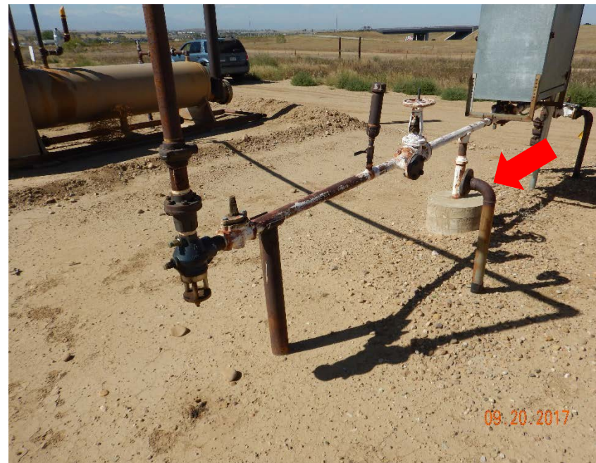
Photo #12 – Uncapped flowline riser on east side of meter run.
