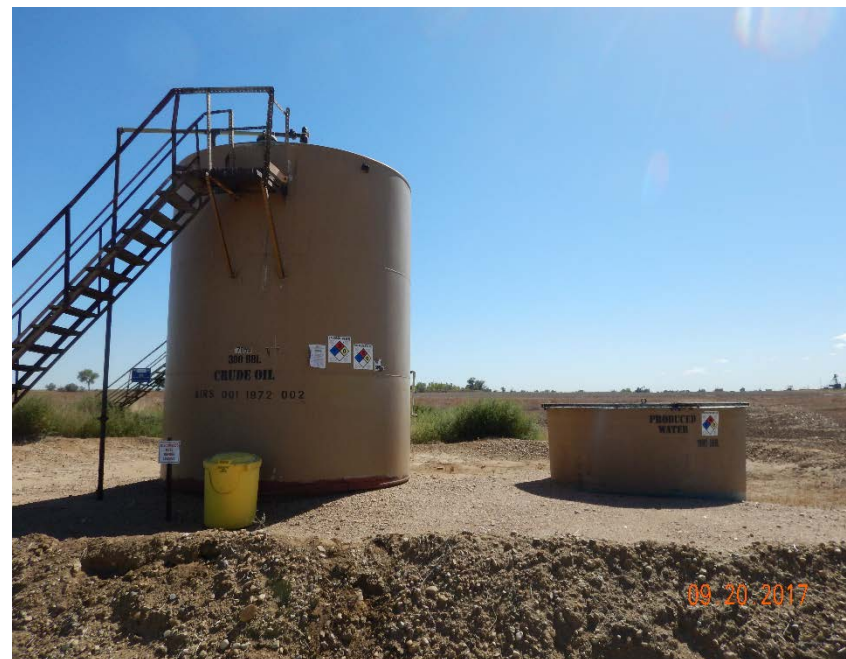
Photo #6 – Tanks with shallow earthen berm.
