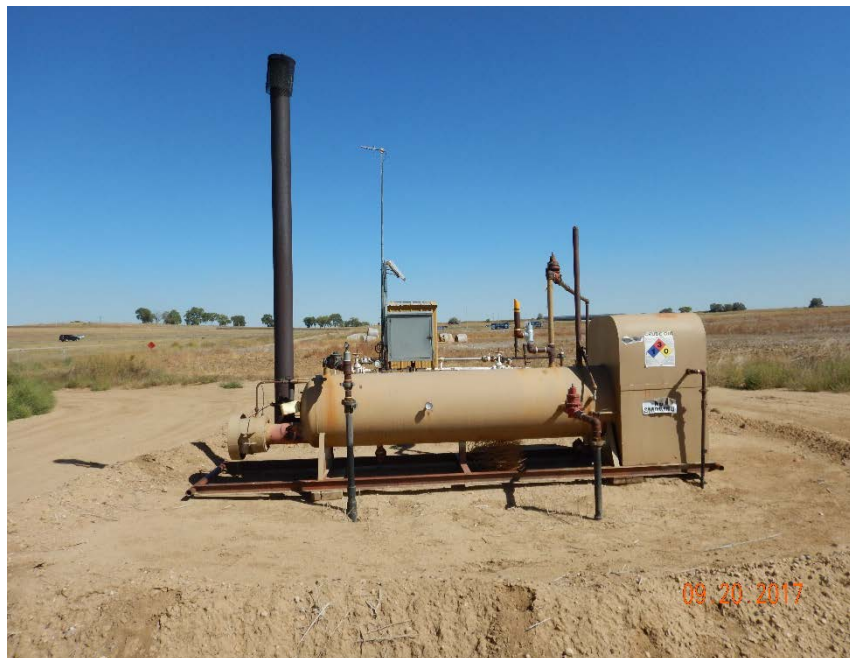
Photo #11 – Horizontal separator with bird protection.
