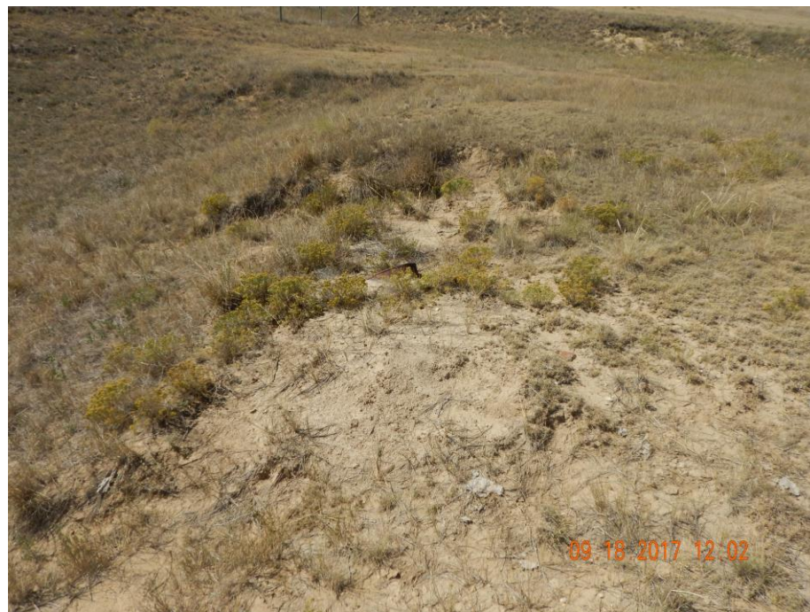
Photo 2: Photo taken from the east end of the pad location. Photo shows erosion degradation due to stormwater runoff. These areas need to be reclaimed.
