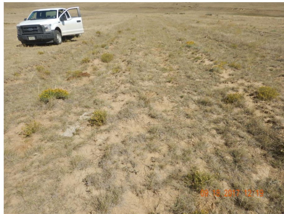
Photo 6: Photo taken from the access road. Photo shows areas of the access road where ruts remain and erosion degradation has occurred. These areas will need to be reclaimed.
