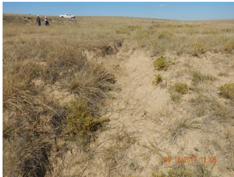
Photo 4: Photo taken from the east end of the pad location, facing northwest. Photo shows erosion degradation due to stormwater runoff. These areas need to be reclaimed.
