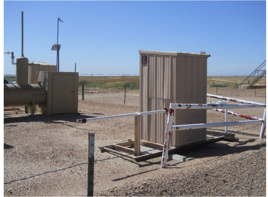
Unused/disconnected gas meter run north of separator
