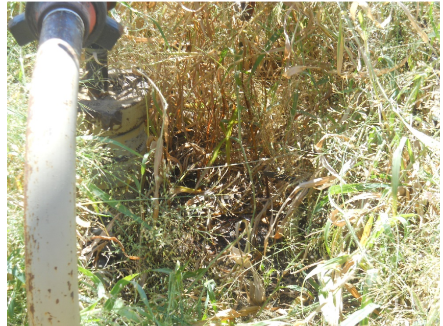
Stained soil under master valve
