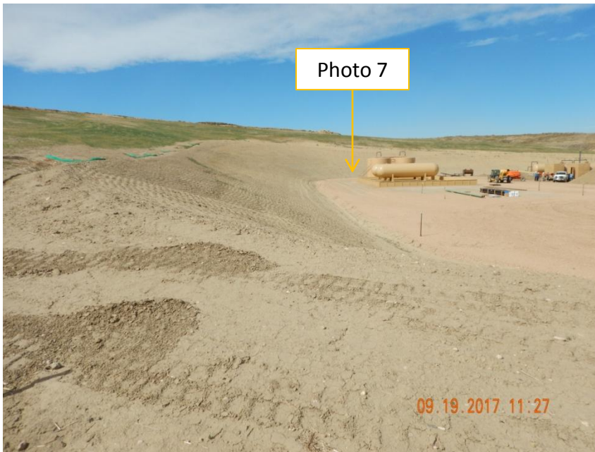
Photo 6. Photo taken from the eastern location, facing West. A perimeter ditch has been installed around the top of the cut slope in conjunction with filtrex wattles to control stormwater run-on. Cut slopes have been temporarily tracked with equipment. Rill erosion was observed along portions of the cut slope- see Photo 7.
