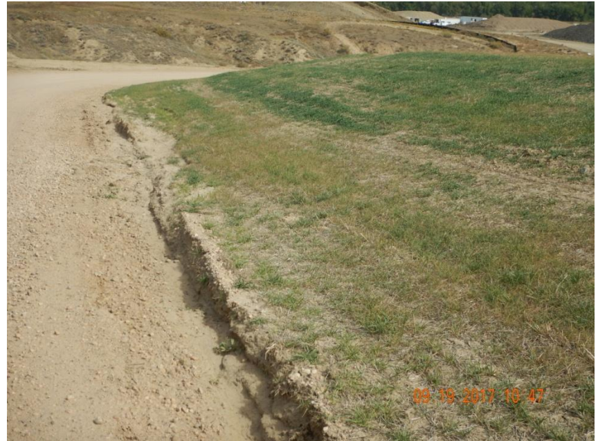
Photo 10. Photo taken from the western location, facing North. Stormwater appears to be travel along the western fill slope and lease road which then runs onto the northwestern location- see Photos 11 & 12.
