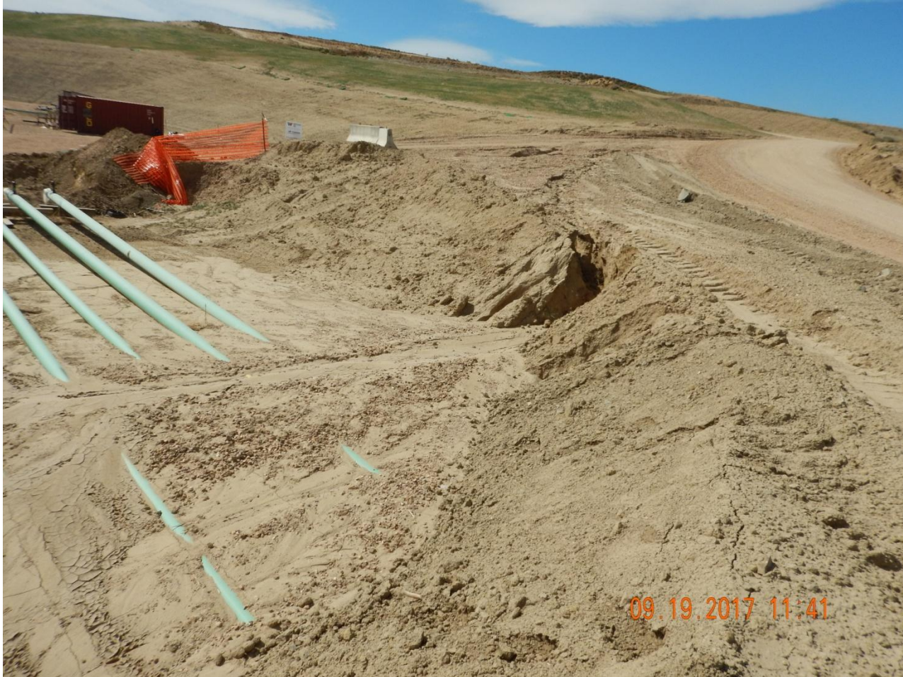
Photo 12. Photo taken from the northwestern location, facing Southwest. Photo illustrates gully and rill erosion occurring along the northwestern location.
