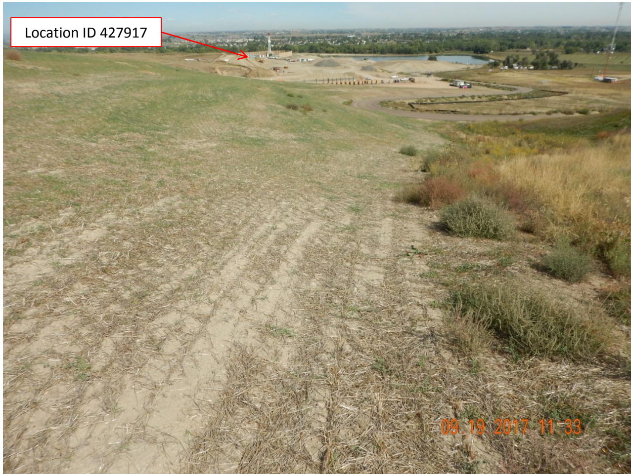
Photo 8. Photo taken from the southern location, facing North. The well pad (Location ID 427917) can be seen in the above photo. Areas constructed to be a berm, as mentioned in Photo 2, do not have uniform germination but appear to be temporarily stabilized with mulch. May need additional reclamation activities for long-term self-sustaining stabilization.
