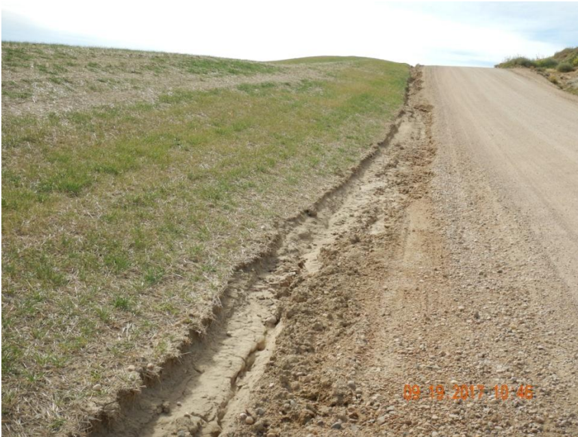
Photo 9. Photo taken from the western location, facing South. Stormwater appears to be travel along the western fill slope and lease road which then runs onto the northwestern location- see Photos 11 & 12.
