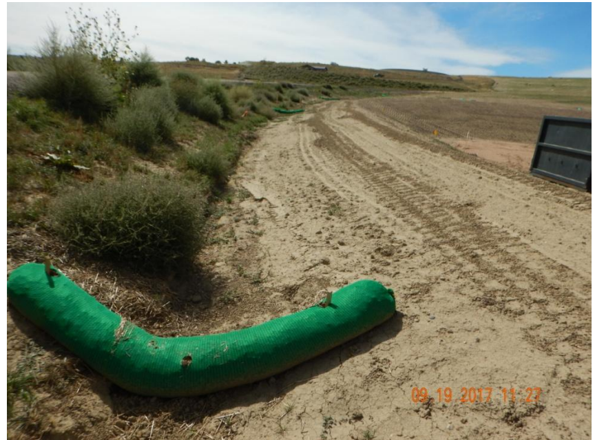
Photo 5. Photo taken from the northeastern pad location, facing South. A perimeter ditch has been installed around the toe of the cut slope in conjunction with filter wattle which is directed to a sediment basin along the northeastern location. Russian thistle and Kochia were observed along the perimeter of the location which needs to be controlled and managed per Rule 603.f.
