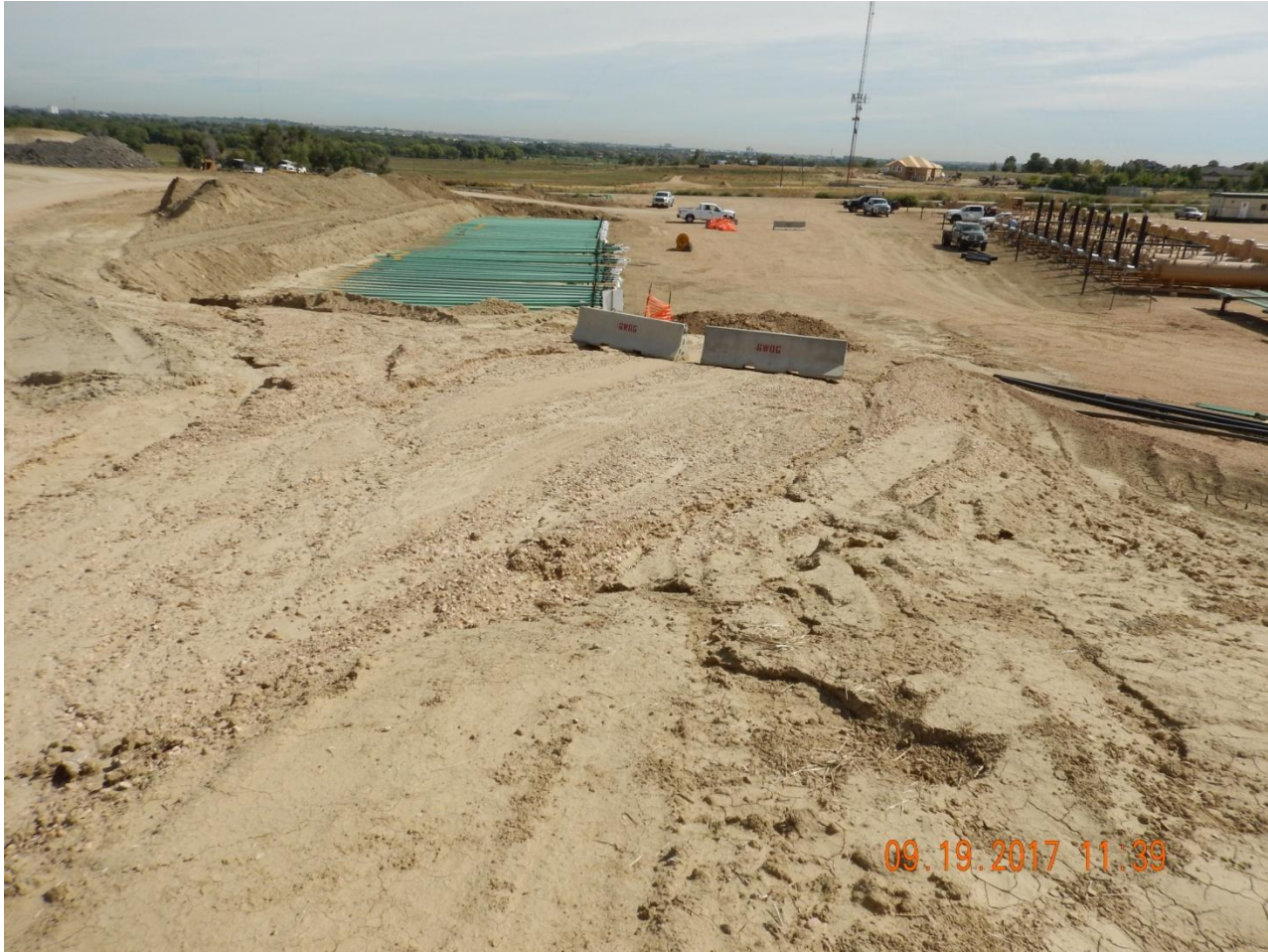
Photo 11. Photo taken from the northwestern location, facing East. Photo illustrates stormwater erosion traveling from the lease road onto location.
