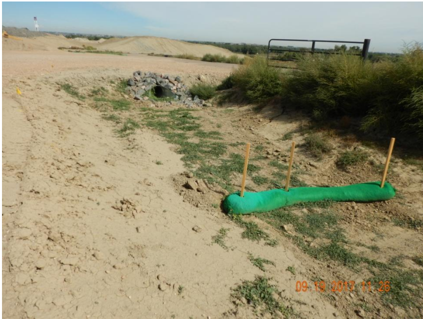
Photo 4. Photo taken from the northeastern pad location, facing North. A perimeter ditch has been installed around the toe of the cut slope in conjunction with filter wattle which is directed to a sediment basin along the northeastern location. Russian thistle and Kochia were observed along the perimeter of the location which needs to be controlled and managed per Rule 603.f.
