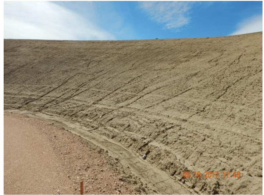
Photo 7. Photo taken from the southwestern pad location, facing South. Rill erosion observed along the western, southwestern and southern cut slope areas. Operator needs to stabilize cut slopes per Rule 1002.f.(2)C.
