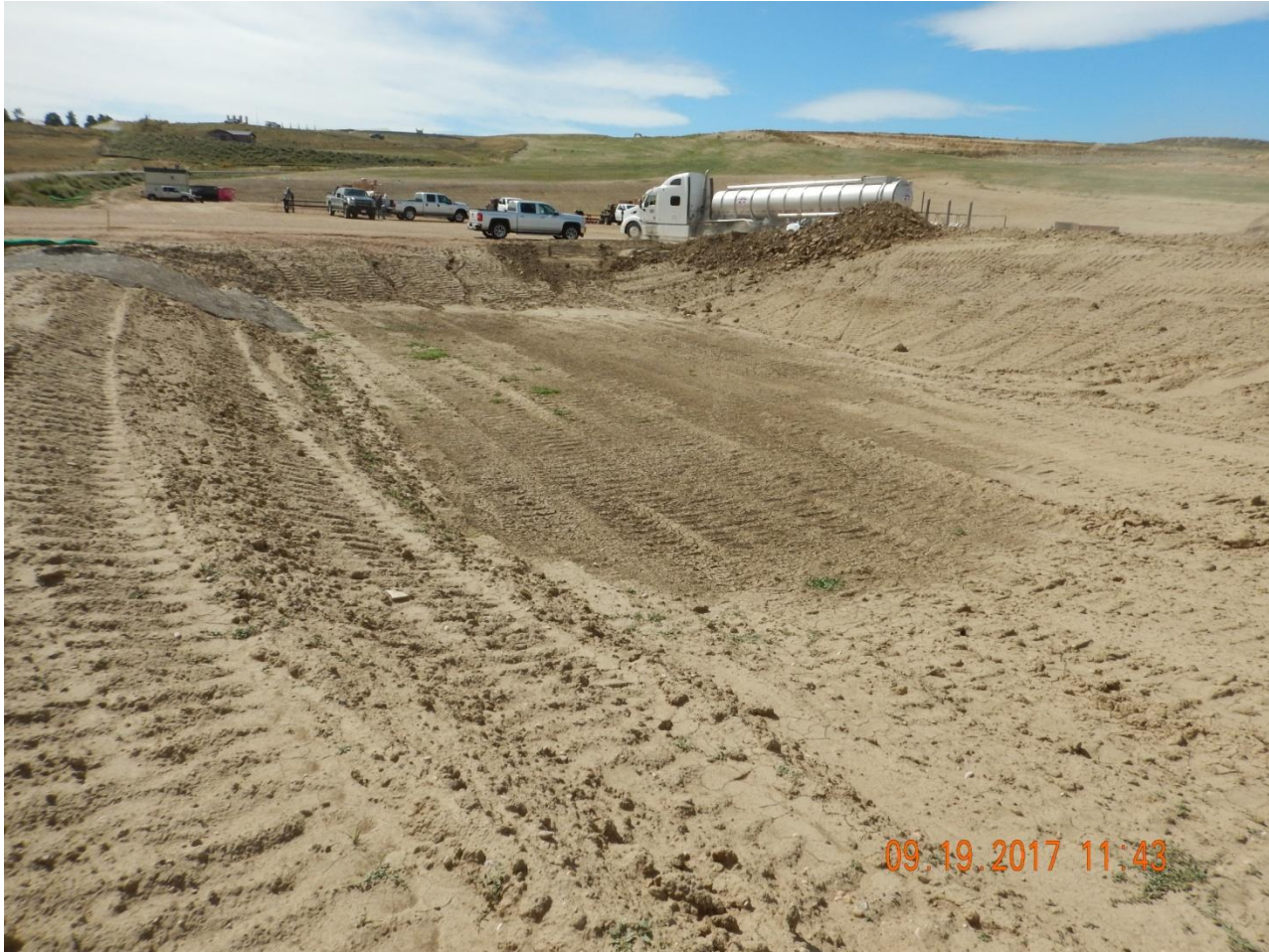
Photo 13. Photo taken from the northeastern location, facing South. Sediment basin has been installed with a stabilized outlet in conjunction with other stormwater BMPs. The sediment basin is downgradient from run-on erosion illustrated in Photos 11 & 12.
