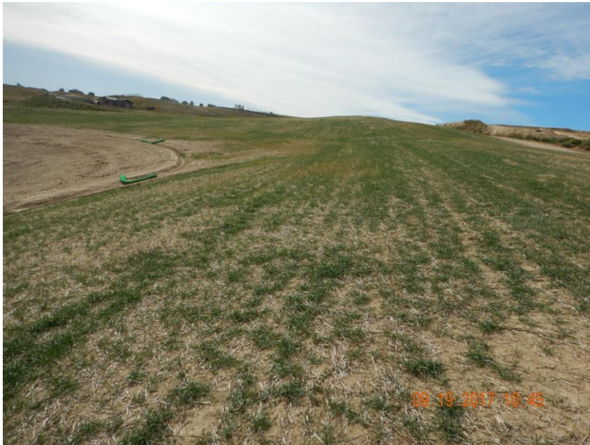
Photo 2. Photo taken from the western location, facing South. The topsoil stockpile has been stored along a portion of the western location. Both the topsoil stockpile and other areas constructed to be a berm have been seeded and mulched. Operator indicated that a “TOPSOIL” sign would be placed to indicate the location of the topsoil.
