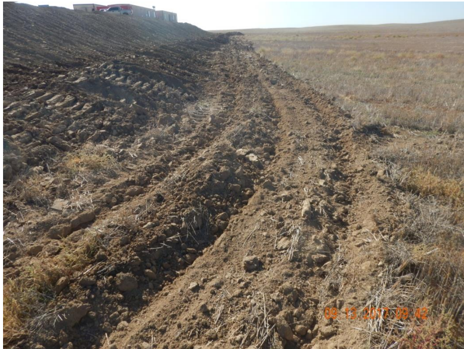
Photo 3: Photo taken from the west end of the location, facing south. Photo shows surface roughening has been implemented along the perimeter of the location.
