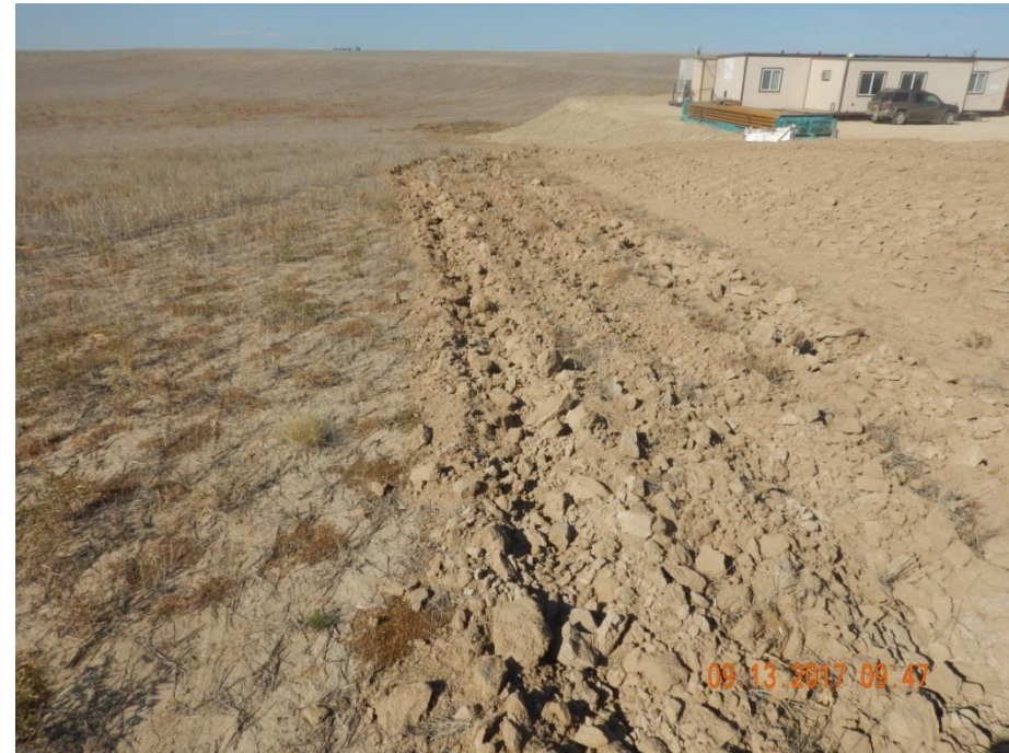
Photo 8: Photo taken from the south end of the location, facing west. Photo shows surface roughening surface had been implemented up the slope, rather than along the contour per good engineering practices. This will likely contribute to erosion and degradation during a stormwater event. Advise implementing additional BMPs to be used in conjunction to surface roughening on the slopes.
