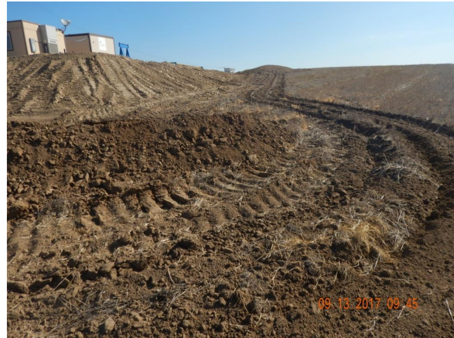
Photo 6: Photo taken from the southwest end of the location, facing east. Please note that surface roughening surface had been implemented up the slope, rather than along the contour per good engineering practices. This will likely contribute to erosion and degradation during a stormwater event. Advise implementing additional BMPs to be used in conjunction to surface roughening on the slopes.
