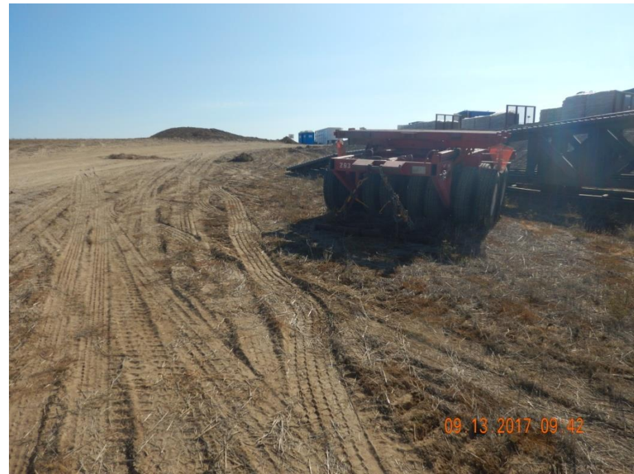
Photo 2: Photo taken from the northeast end of the location, facing east. North and south ends of location along slope of hill. Areas of the access road and north end of the location at risk to stormwater degradation. Advise incorporating additional BMPs in these areas.
