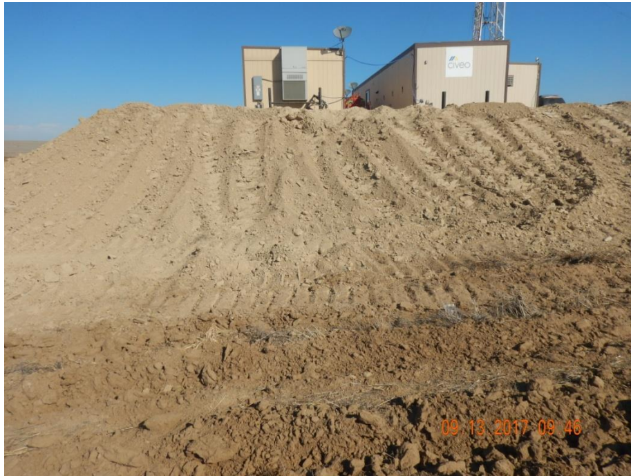
Photo 7: Photo taken from the south end of the location, facing north. Photo shows tracking had been attempted on the slopes, however slopes remain largely un-consolidated.
