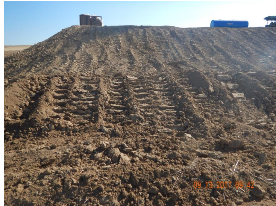
Photo 4: Photo taken from the west end of the location, facing east. Photo shows slopes of the pad and berms have been tracked, but remain largely unconsolidated. In their current condition BMPs are sufficient on a temporary basis, however slopes and berms will require additional consolidation once more permanent BMPs are required.
