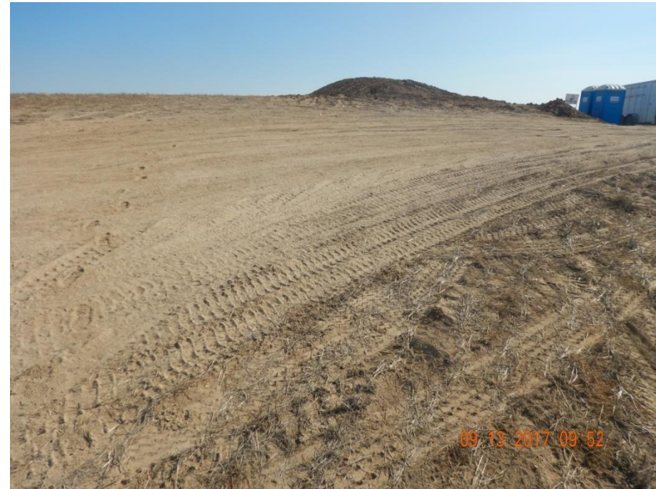
Photo 14: Photo taken from the north end of the location, facing east. Photo shows areas of the access road and north end of the location at risk to stormwater degradation. Advise incorporating additional BMPs in these areas.
