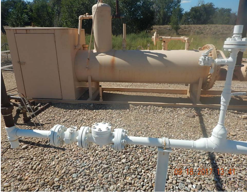
Photo 6: Separator improperly anchored.
