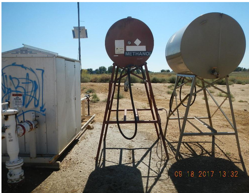
Photo 5 Methanol Tanks (Note, tank on right is labeled DCP)
