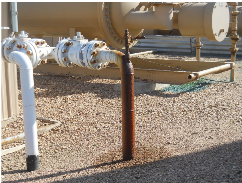
Leaking valve at gas meter run that is staining soil.
