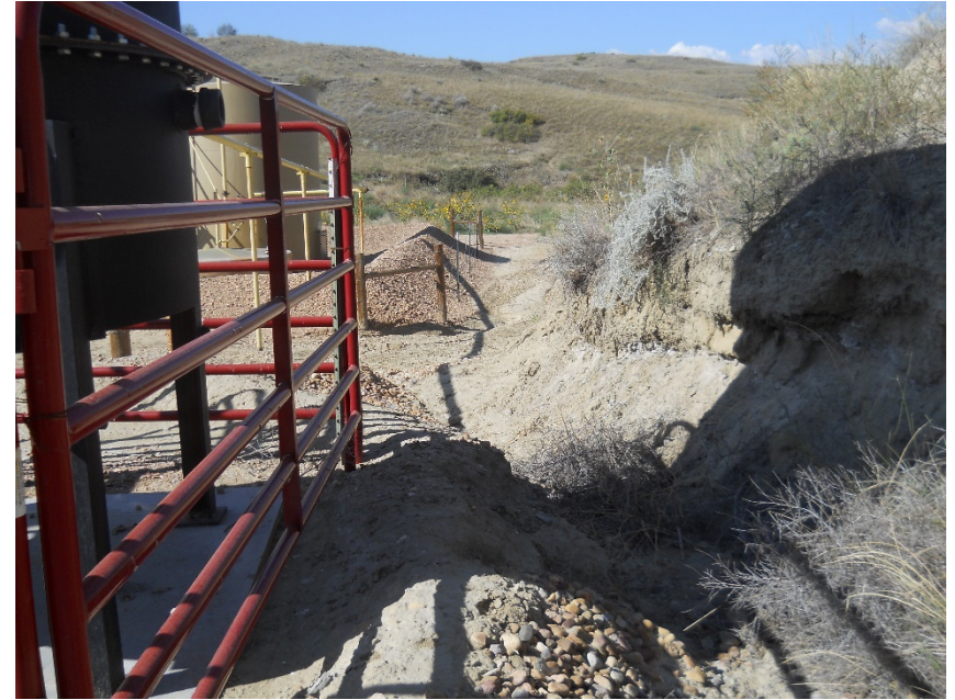
Location washing out north side of location, discharging northwest of tank battery with sediment carrying off into field
