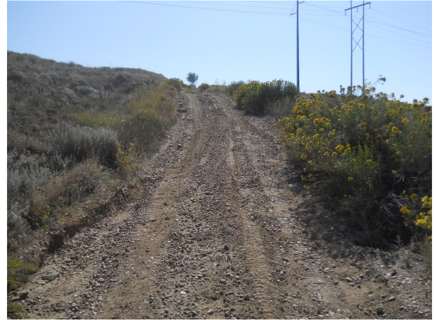
Access road to wellhead from battery looking southeast. Road is washing out on both sides
