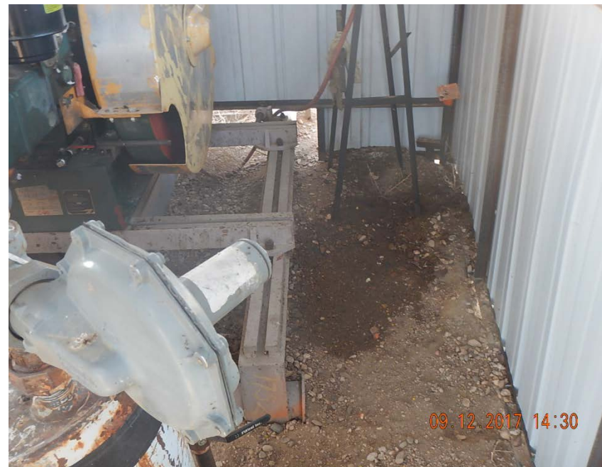
Photo 6: Stained soil at engine
