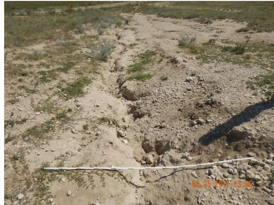
Photo 7: Photo taken from the northeast of pit/location, facing east. Photo shows stormwater runoff from the location has caused erosion degradation on the adjacent lands. Erosion will need to be repaired and stabilized. Required BMPs will need to be installed and maintained in accordance to 1002.f to prevent further degradation. These areas will need to be re-vegetated/reclaimed. Soil testing is advised as contaminants may exist preventing vegetation from re-establishing.
