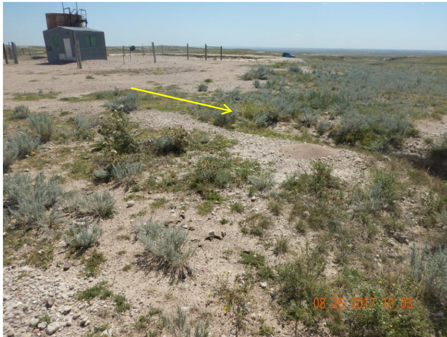
Photo 2: Photo taken from the west end of the location, facing south. Photo shows gully formation on the west end of the location.
