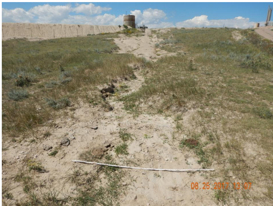
Photo 12: Photo taken east of the location, facing east. Photo shows stormwater runoff from the location has caused erosion degradation on the adjacent lands. Erosion will need to be repaired and stabilized. Required BMPs will need to be installed and maintained in accordance to 1002.f to prevent further degradation. These areas will need to be re-vegetated/reclaimed. Soil testing is advised as contaminants may exist preventing vegetation from re-establishing.
