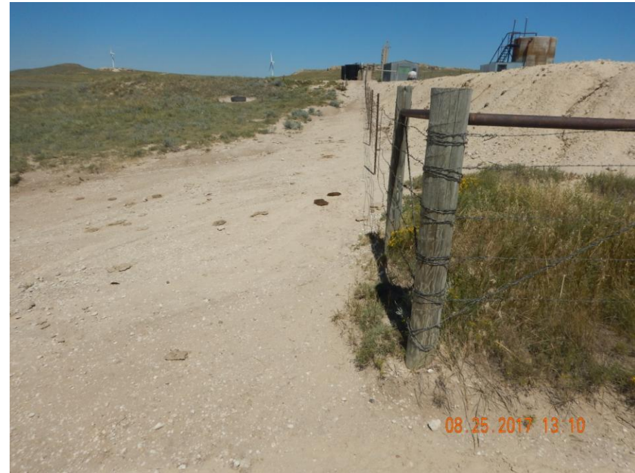
Photo 19: Photo taken on the south end of the location, facing northeast. Photo shows stormwater runoff from the location has caused erosion degradation on the adjacent lands. Erosion will need to be repaired and stabilized. Required BMPs will need to be installed and maintained in accordance to 1002.f to prevent further degradation. These areas will need to be re-vegetated/reclaimed. Soil testing is advised as contaminants may exist preventing vegetation from re-establishing.
