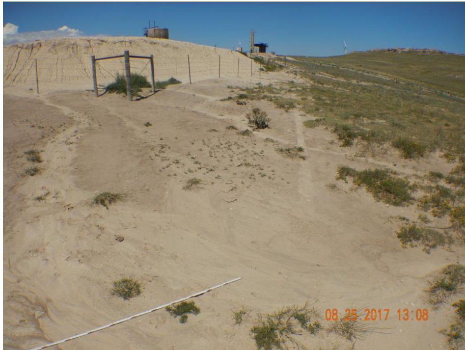
Photo 16: Photo taken from the southeast end of the pit, facing north. Photo shows stormwater runoff from the location has caused erosion degradation on the adjacent lands. Erosion will need to be repaired and stabilized. Required BMPs will need to be installed and maintained in accordance to 1002.f to prevent further degradation. These areas will need to be re-vegetated/reclaimed. Soil testing is advised as contaminants may exist preventing vegetation from re-establishing.
