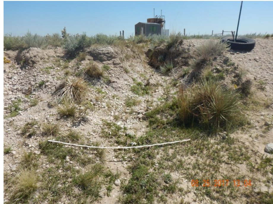
Photo 5: Photo taken from the west end of the location, facing east. Photo shows gully formation due to stormwater erosion from the location. Erosion will need to be repaired and stabilized. Required BMPs will need to be installed and maintained in accordance to 1002.f to prevent further degradation. 6 foot measuring stick for reference.
