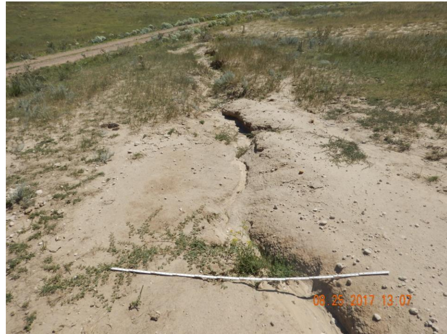
Photo 11: Photo taken east of the location, facing east. Photo shows stormwater runoff from the location has caused erosion degradation on the adjacent lands. Erosion will need to be repaired and stabilized. Required BMPs will need to be installed and maintained in accordance to 1002.f to prevent further degradation. These areas will need to be re-vegetated/reclaimed. Soil testing is advised as contaminants may exist preventing vegetation from re-establishing.
