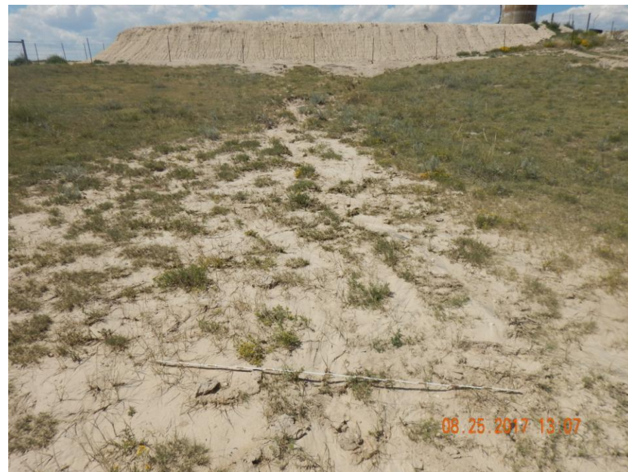
Photo 13: Photo taken east of the location, facing east. Photo shows stormwater runoff from the location has caused erosion degradation on the adjacent lands. Erosion will need to be repaired and stabilized. Required BMPs will need to be installed and maintained in accordance to 1002.f to prevent further degradation. These areas will need to be re-vegetated/reclaimed. Soil testing is advised as contaminants may exist preventing vegetation from re-establishing.
