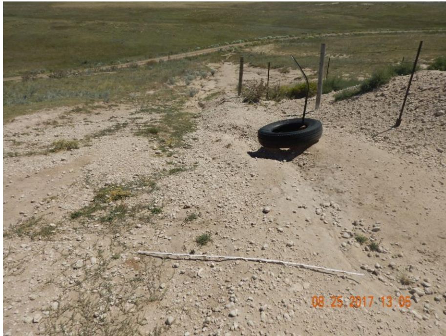
Photo 6: Photo taken on the east end of the location, facing east. Photo shows degradation on location due to stormwater erosion. Erosion will need to be repaired and stabilized. Required BMPs will need to be installed and maintained in accordance to 1002.f to prevent further degradation. These areas will need to be re-vegetated/reclaimed. Soil testing is advised as contaminants may exist preventing vegetation from re-establishing. 6 foot measuring stick for reference.
