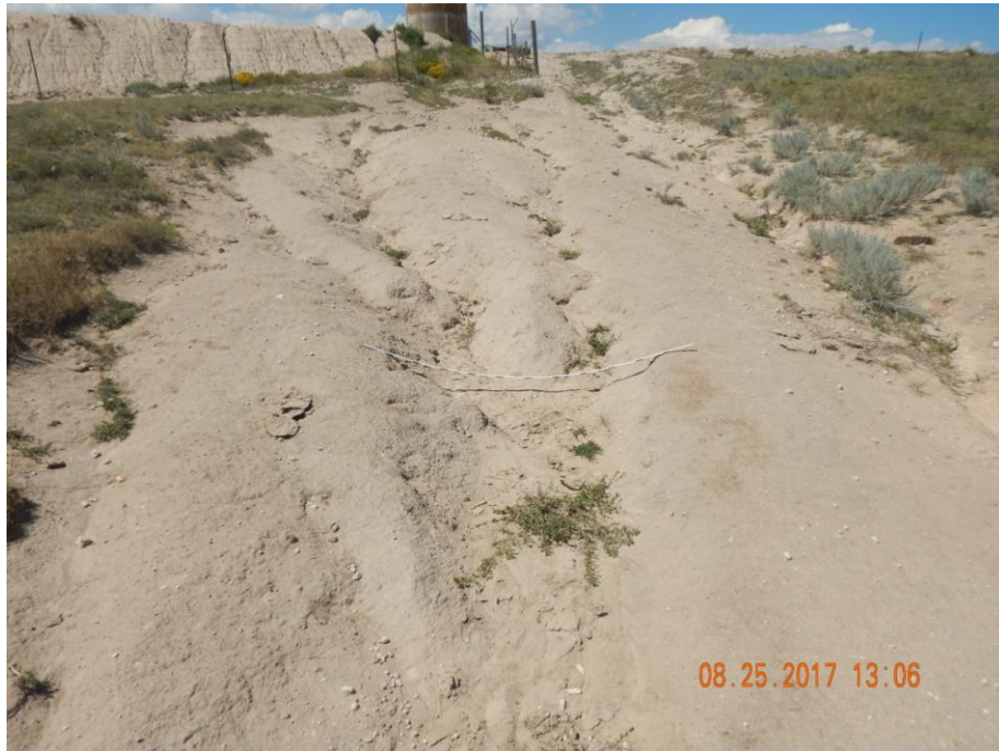
Photo 10: Photo taken east of the location, facing west. Photo shows stormwater runoff from the location has caused erosion degradation on the adjacent lands. Erosion will need to be repaired and stabilized. Required BMPs will need to be installed and maintained in accordance to 1002.f to prevent further degradation. These areas will need to be re-vegetated/reclaimed. Soil testing is advised as contaminants may exist preventing vegetation from re-establishing.
