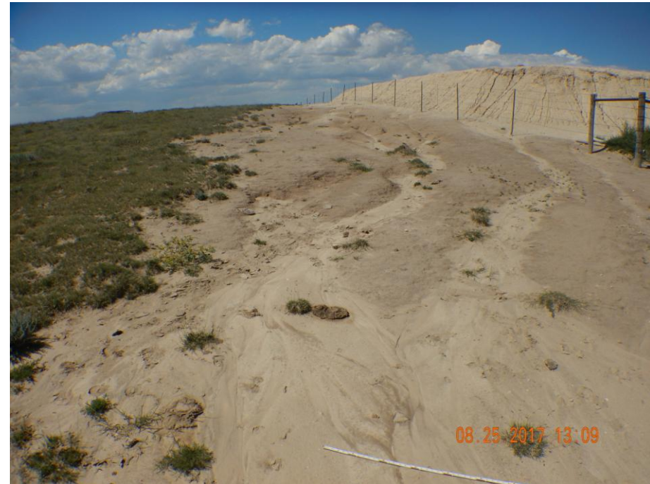
Photo 17: Photo taken from the southeast end of the pit, facing north. Photo shows stormwater runoff from the location has caused erosion degradation on the adjacent lands. Erosion will need to be repaired and stabilized. Required BMPs will need to be installed and maintained in accordance to 1002.f to prevent further degradation. These areas will need to be re-vegetated/reclaimed. Soil testing is advised as contaminants may exist preventing vegetation from re-establishing.
