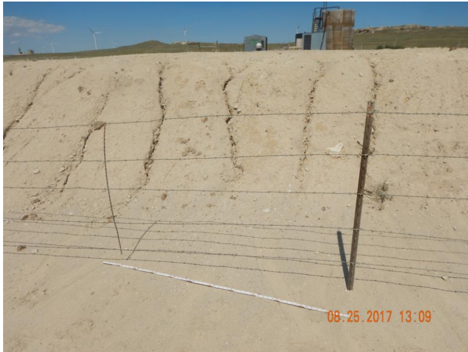
Photo 18: Photo taken on the south end of the pit. Photo shows rill erosion formations on the berms of the pit caused by stormwater.
