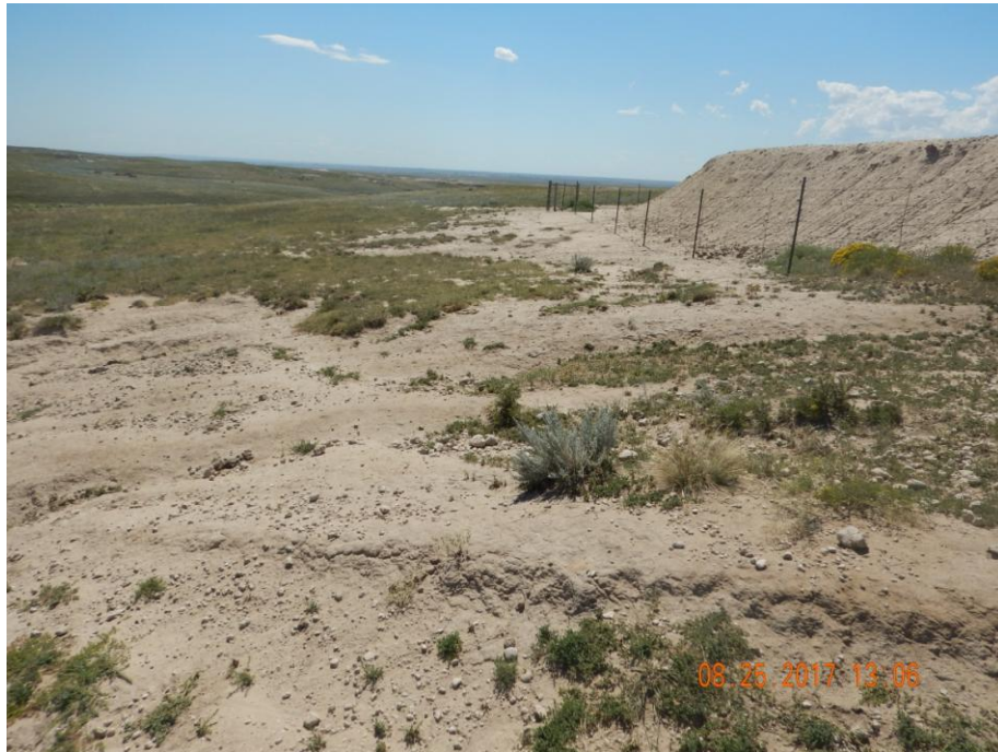
Photo 8: Photo taken on the east end of the location, facing south. Photo shows stormwater runoff from the location has caused erosion degradation on the adjacent lands. Erosion will need to be repaired and stabilized. Required BMPs will need to be installed and maintained in accordance to 1002.f to prevent further degradation. These areas will need to be re-vegetated/reclaimed. Soil testing is advised as contaminants may exist preventing vegetation from re-establishing.
