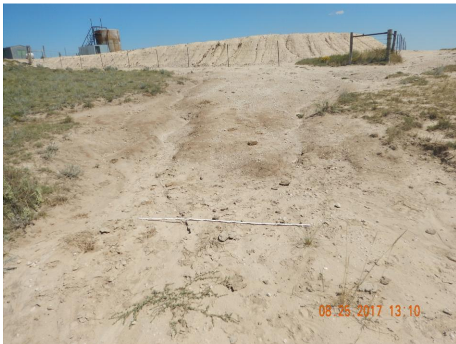
Photo 20: Photo taken from the southwest of the pit, facing northeast. Photo shows stormwater runoff from the location has caused erosion degradation on the adjacent lands. Erosion will need to be repaired and stabilized. Required BMPs will need to be installed and maintained in accordance to 1002.f to prevent further degradation. These areas will need to be re-vegetated/reclaimed. Soil testing is advised as contaminants may exist preventing vegetation from re-establishing.
