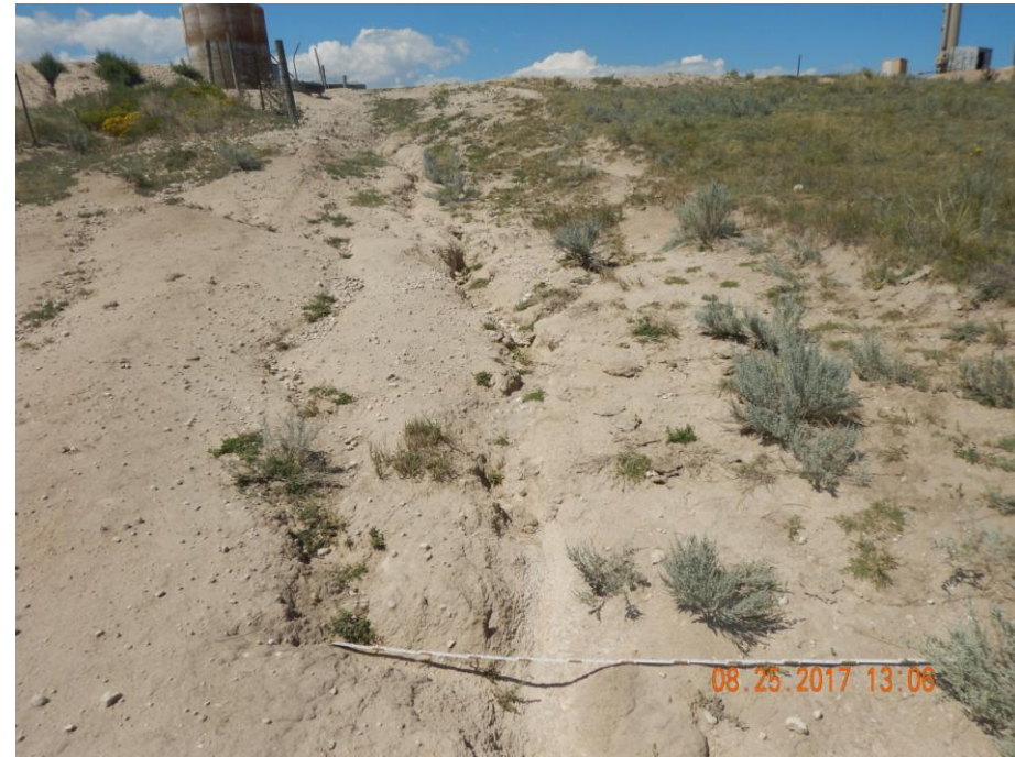
Photo 9: Photo taken east of the location, facing west. Photo shows stormwater runoff from the location has caused erosion degradation on the adjacent lands. Erosion will need to be repaired and stabilized. Required BMPs will need to be installed and maintained in accordance to 1002.f to prevent further degradation. These areas will need to be re-vegetated/reclaimed. Soil testing is advised as contaminants may exist preventing vegetation from re-establishing.
