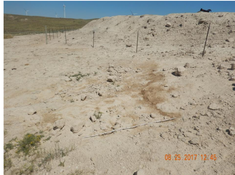
Photo 19: Photo taken on the southwest corner of the pit, facing north. Photo shows stormwater runoff and erosion degradation occurring at the pit. Runoff from the location has caused erosion degradation on the adjacent lands. Erosion will need to be repaired and stabilized. Required BMPs will need to be installed and maintained in accordance to 1002.f to prevent further degradation. These areas will need to be re-vegetated/reclaimed. Erosion evident as far back, and likely prior to, 1998 (see photo 6b); soil testing is advised as contaminants may exist preventing vegetation from re-establishing. 6 foot measuring stick for reference.
