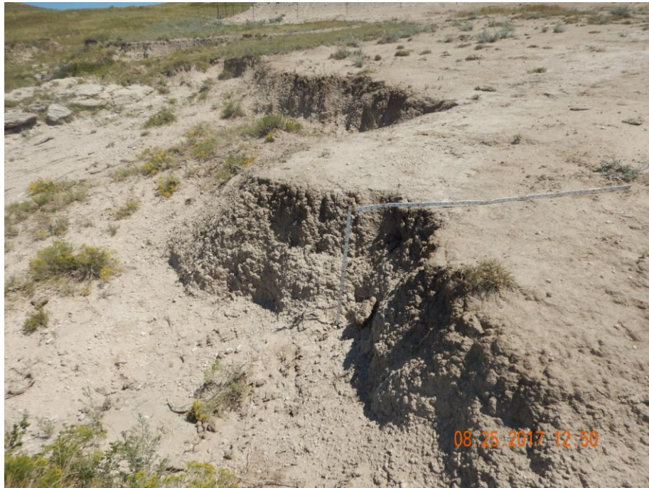
Photo 30: Photo taken from the west of the pit, facing north. Photo shows large headcuts have formed due to stormwater erosion from the location. Headcut seen here is ~2 feet in height. There are other headcuts in the area that appear to be larger in size.
