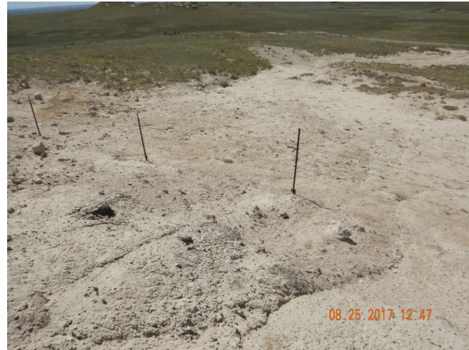
Photo 23: Photo taken on the west end of the pit, facing southwest. Photo shows stormwater runoff from the location has caused erosion degradation on the adjacent lands. Erosion will need to be repaired and stabilized. Required BMPs will need to be installed and maintained in accordance to 1002.f to prevent further degradation. These areas will need to be re-vegetated/reclaimed. Erosion evident as far back, and likely prior to, 1998 (see photo 6b); soil testing is advised as contaminants may exist preventing vegetation from re-establishing.
