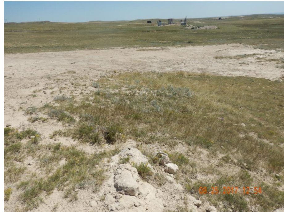
Photo 45: Photo taken from the south end of the pit, facing southeast. Photo shows stormwater runoff from the location has caused erosion degradation on the adjacent lands. Erosion will need to be repaired and stabilized. Required BMPs will need to be installed and maintained in accordance to 1002.f to prevent further degradation. These areas will need to be re-vegetated/reclaimed. Soil testing is advised as contaminants may exist preventing vegetation from re-establishing.
