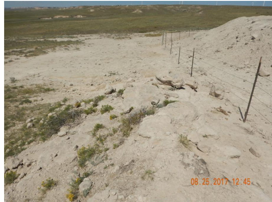
Photo 17: Photo taken on the southwest corner of the pit, facing northwest. Photo shows stormwater runoff from the location has caused erosion degradation on the adjacent lands. Erosion will need to be repaired and stabilized. Required BMPs will need to be installed and maintained in accordance to 1002.f to prevent further degradation. These areas will need to be re-vegetated/reclaimed. Erosion evident as far back, and likely prior to, 1998 (see photo 6b); soil testing is advised as contaminants may exist preventing vegetation from re-establishing.
