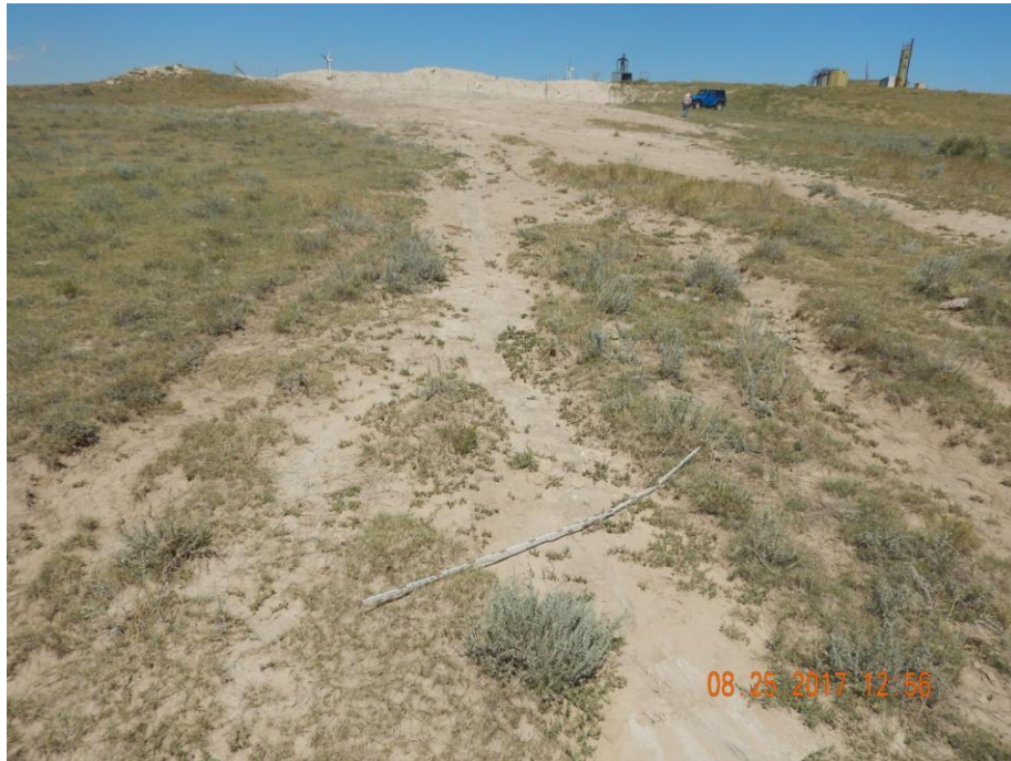
Photo 48: Photo taken from the south of the pit, facing north. Photo shows stormwater runoff from the location has caused erosion degradation on the adjacent lands. Erosion will need to be repaired and stabilized. Required BMPs will need to be installed and maintained in accordance to 1002.f to prevent further degradation. These areas will need to be re-vegetated/reclaimed. Soil testing is advised as contaminants may exist preventing vegetation from re-establishing. 6 foot measuring stick for reference.
