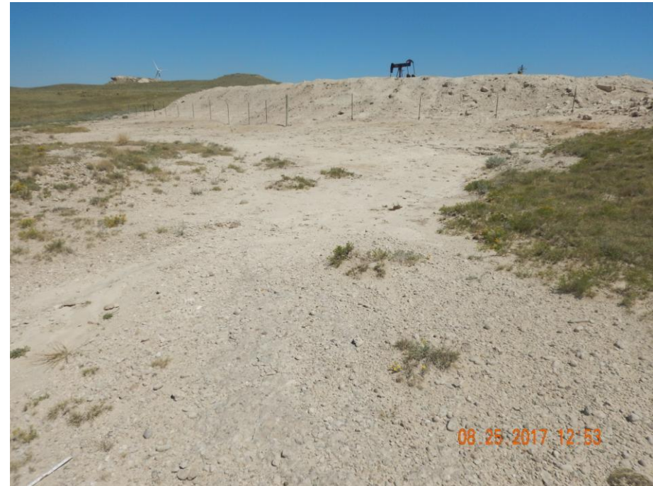
Photo 41: Photo taken from the southwest of the pit, facing northeast. Photo shows stormwater runoff from the location has caused erosion degradation on the adjacent lands. Erosion will need to be repaired and stabilized. Required BMPs will need to be installed and maintained in accordance to 1002.f to prevent further degradation. These areas will need to be re-vegetated/reclaimed. Soil testing is advised as contaminants may exist preventing vegetation from re-establishing.
