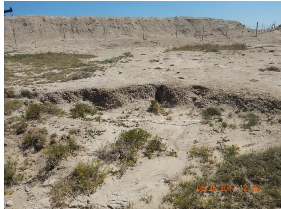
Photo 25: Photo taken from the west of the pit, facing east. Photo shows large headcuts have formed due to stormwater erosion from the location. Erosion will need to be repaired and stabilized. Required BMPs will need to be installed and maintained in accordance to 1002.f to prevent further degradation. These areas will need to be re-vegetated/reclaimed. Erosion evident as far back, and likely prior to, 1998 (see photo 6b); soil testing is advised as contaminants may exist preventing vegetation from re-establishing. 6 foot measuring stick for reference.
