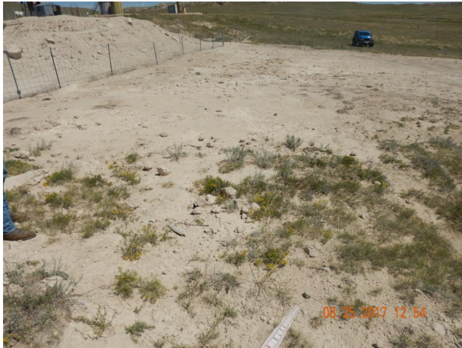
Photo 44: Photo taken from the south end of the pit, facing east. Photo shows stormwater runoff from the location has caused erosion degradation on the adjacent lands. Erosion will need to be repaired and stabilized. Required BMPs will need to be installed and maintained in accordance to 1002.f to prevent further degradation. These areas will need to be re-vegetated/reclaimed. Soil testing is advised as contaminants may exist preventing vegetation from re-establishing.
