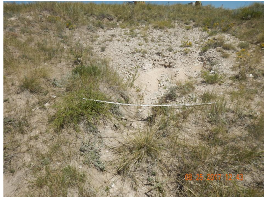
Photo 13: Photo taken on the south end of the location, facing northeast. Photo shows stormwater runoff from the location has caused erosion degradation on the adjacent lands. Erosion will need to be repaired and stabilized. Required BMPs will need to be installed and maintained in accordance to 1002.f to prevent further degradation. 6 foot measuring stick for reference.
