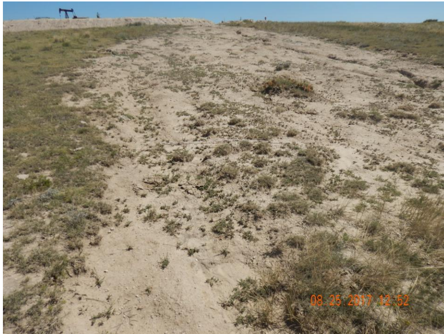
Photo 36: Photo taken from the southwest of the pit, facing north. Photo shows stormwater runoff from the location has caused erosion degradation on the adjacent lands. Erosion will need to be repaired and stabilized. Required BMPs will need to be installed and maintained in accordance to 1002.f to prevent further degradation. These areas will need to be re-vegetated/reclaimed. Soil testing is advised as contaminants may exist preventing vegetation from re-establishing. 6 foot measuring stick for reference.
