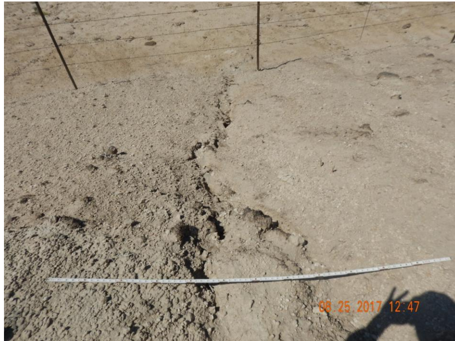
Photo 24: Photo taken from the west end of the pit. Photo shows stormwater runoff and erosion degradation occurring at the pit. Runoff from the location has caused erosion degradation on the adjacent lands. Erosion will need to be repaired and stabilized. Required BMPs will need to be installed and maintained in accordance to 1002.f to prevent further degradation. 6 foot measuring stick for reference.
