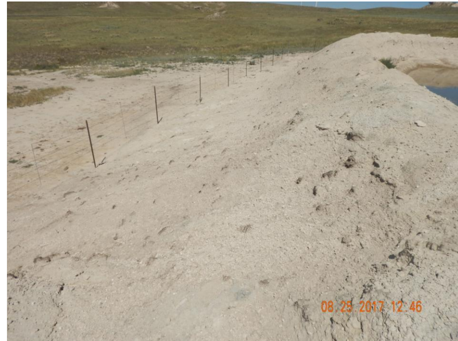
Photo 21: Photo taken on the west end of the pit, facing north. Photo shows stormwater runoff from the location has caused erosion degradation on the adjacent lands. Erosion will need to be repaired and stabilized. Required BMPs will need to be installed and maintained in accordance to 1002.f to prevent further degradation. These areas will need to be re-vegetated/reclaimed. Erosion evident as far back, and likely prior to, 1998 (see photo 6b); soil testing is advised as contaminants may exist preventing vegetation from re-establishing.
