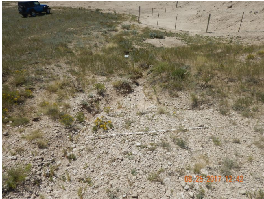
Photo 12: Photo taken on the south end of the location, facing southwest. Photo shows stormwater runoff from the location has caused erosion degradation on the adjacent lands. Erosion will need to be repaired and stabilized. Required BMPs will need to be installed and maintained in accordance to 1002.f to prevent further degradation. 6 foot measuring stick for reference.
