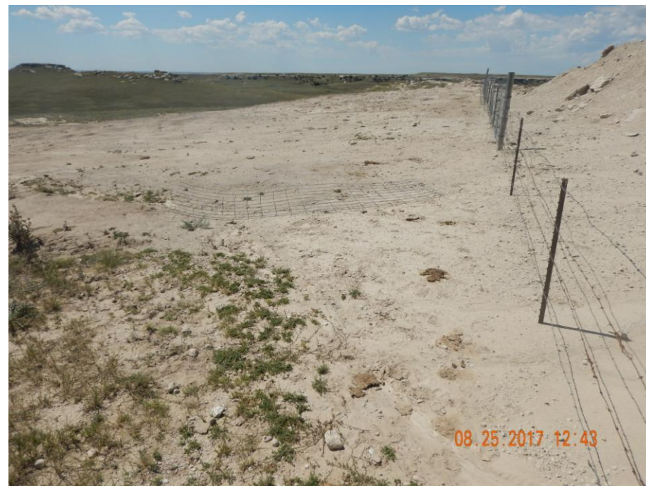
Photo 15: Photo taken on the southeast corner of the pit, facing west. Photo shows stormwater runoff from the location has caused erosion degradation on the adjacent lands. Erosion will need to be repaired and stabilized. Required BMPs will need to be installed and maintained in accordance to 1002.f to prevent further degradation. These areas will need to be re-vegetated/reclaimed. Erosion evident as far back, and likely prior to, 1998 (see photo 6b); soil testing is advised as contaminants may exist preventing vegetation from re-establishing.
