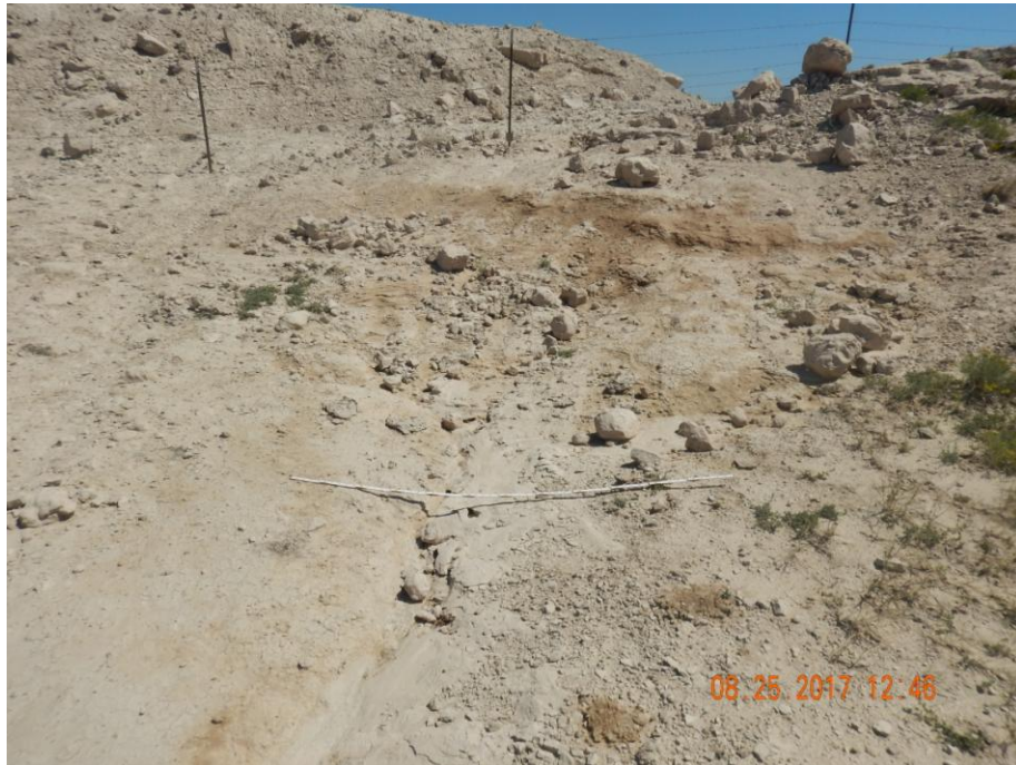
Photo 20: Photo taken on the southwest corner of the pit, facing northeast. Photo shows stormwater runoff and erosion degradation occurring at the pit. Runoff from the location has caused erosion degradation on the adjacent lands. Erosion will need to be repaired and stabilized. Required BMPs will need to be installed and maintained in accordance to 1002.f to prevent further degradation. These areas will need to be re-vegetated/reclaimed. Erosion evident as far back, and likely prior to, 1998 (see photo 6b); soil testing is advised as contaminants may exist preventing vegetation from re-establishing. 6 foot measuring stick for reference.
