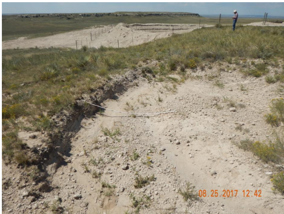
Photo 10: Photo taken on the south end of the location, facing west. Photo shows degradation on location due to stormwater erosion. Erosion will need to be repaired and stabilized. Required BMPs will need to be installed and maintained in accordance to 1002.f to prevent further degradation. 6 foot measuring stick for reference.
