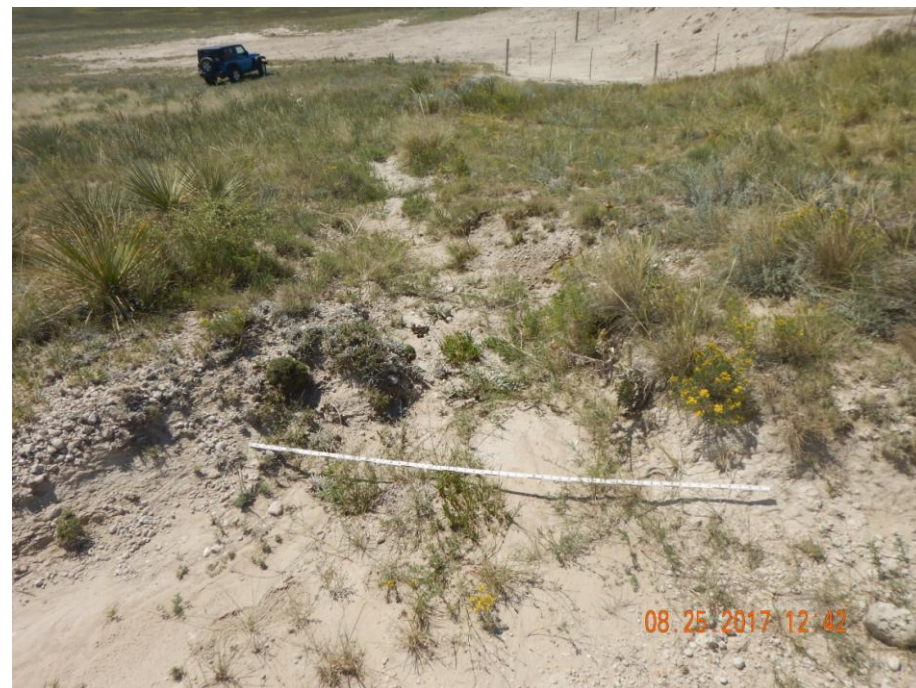
Photo 11: Photo taken on the south end of the location, facing southwest. Photo shows stormwater runoff from the location has caused erosion degradation on the adjacent lands. Erosion will need to be repaired and stabilized. Required BMPs will need to be installed and maintained in accordance to 1002.f to prevent further degradation. 6 foot measuring stick for reference.
