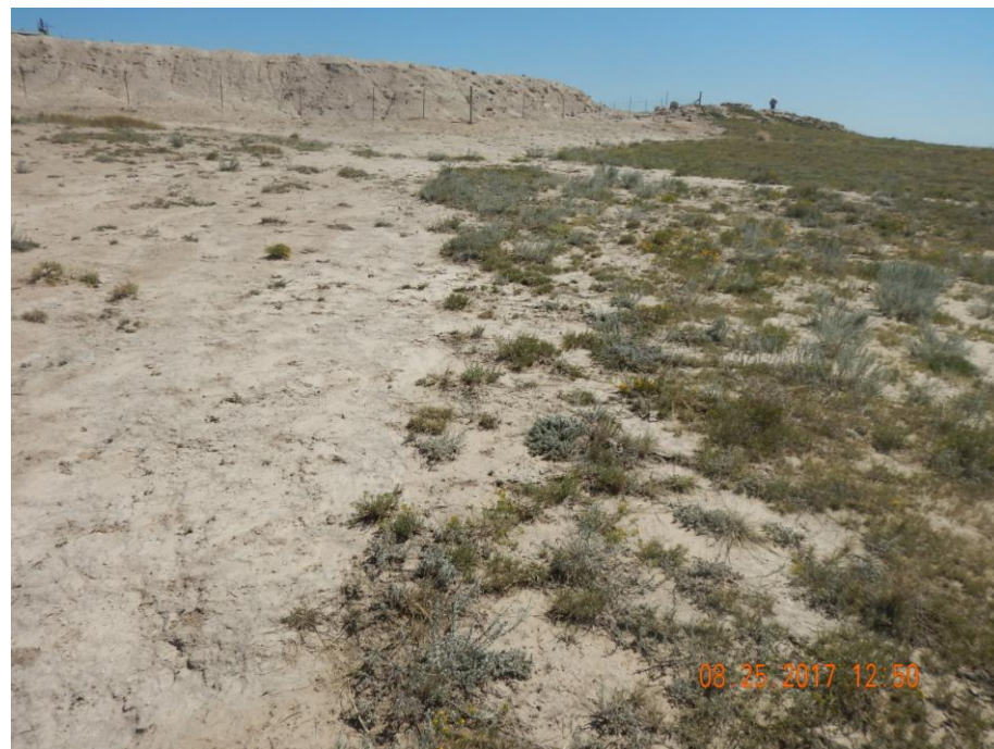
Photo 33: Photo taken from the southwest of the pit, facing east. Photo shows stormwater runoff from the location has caused erosion degradation on the adjacent lands. Erosion will need to be repaired and stabilized. Required BMPs will need to be installed and maintained in accordance to 1002.f to prevent further degradation. These areas will need to be re-vegetated/reclaimed. Soil testing is advised as contaminants may exist preventing vegetation from re-establishing.
