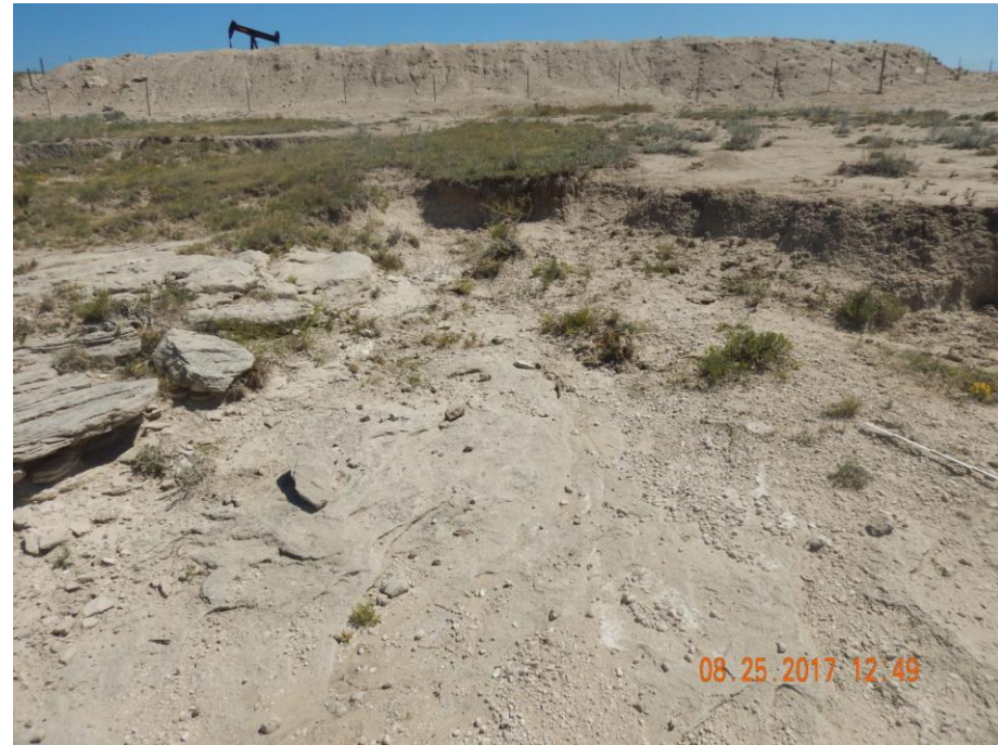
Photo 29: Photo taken from the west of the pit, facing east. Photo shows large headcuts have formed due to stormwater erosion from the location. Erosion will need to be repaired and stabilized. Required BMPs will need to be installed and maintained in accordance to 1002.f to prevent further degradation. These areas will need to be re-vegetated/reclaimed. Erosion evident as far back, and likely prior to, 1998 (see photo 6b); soil testing is advised as contaminants may exist preventing vegetation from re-establishing. 6 foot measuring stick for reference.
