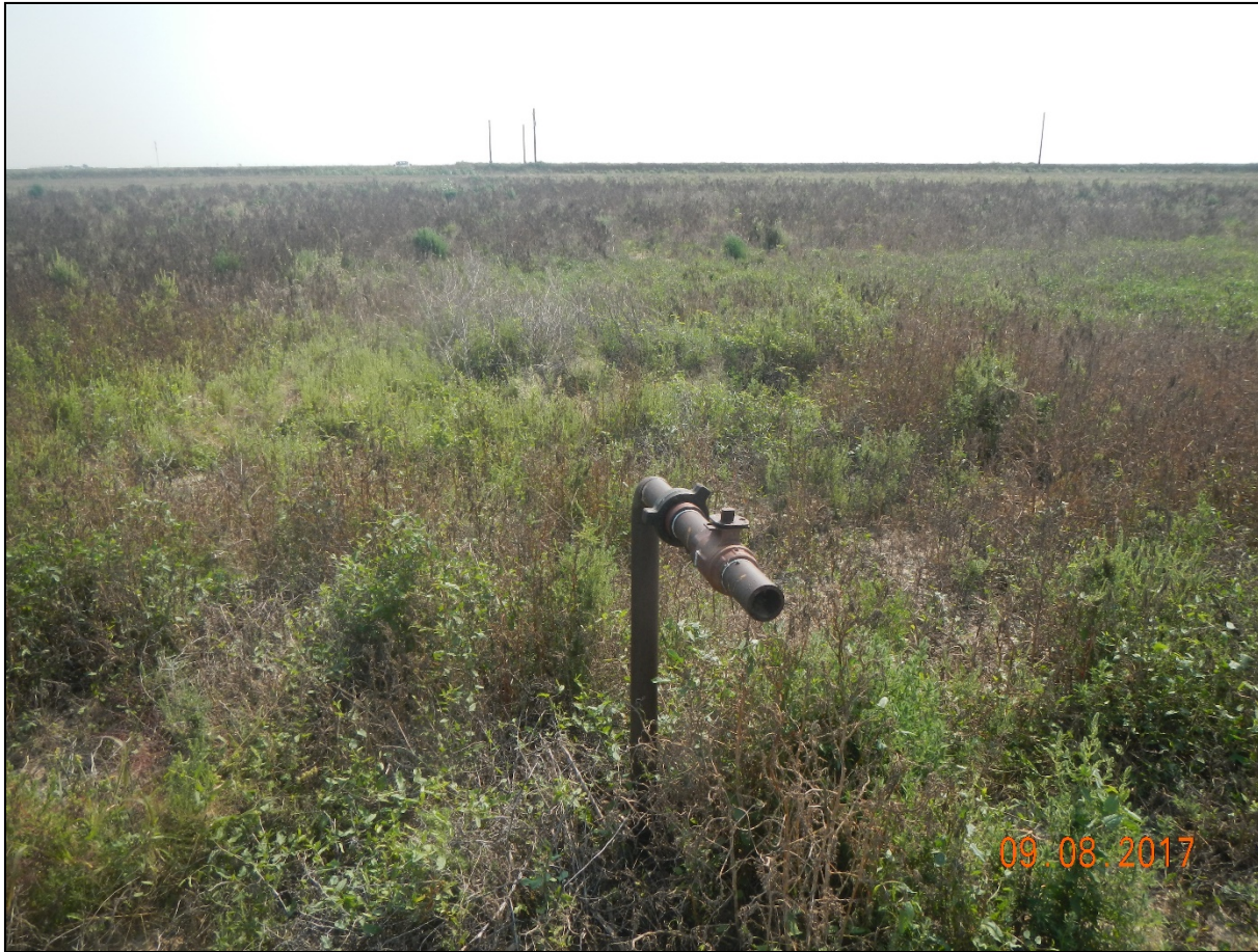
Photo 2. An abandoned pipe riser remains at the location.
