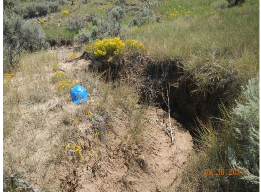
Photo 4: View downstream of headcut in Photo 3, approximately 4 feet wide and 5 feet deep. This needs to be stabilized.
