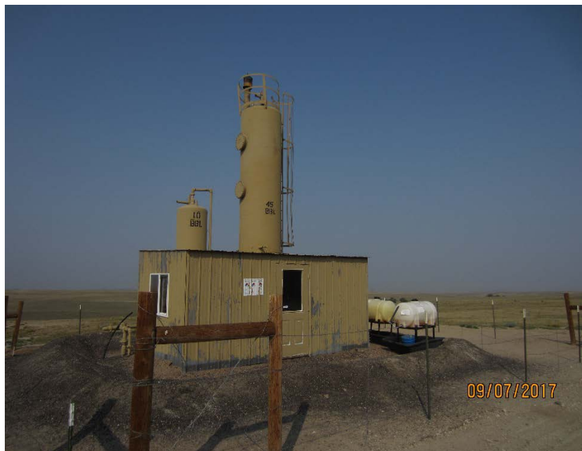
Photo #5 – VHT shed with day tanks inside of berm.
