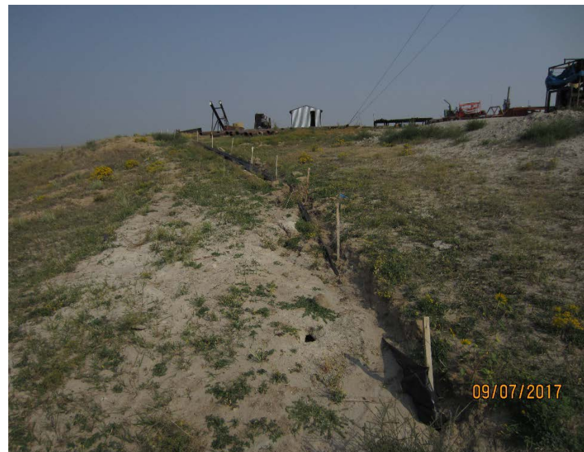
Photo #10 – Southern end of silt fence that runs along west side of location. Silt fence in need of repair/maintenance. Note sediment transport west of silt fence.
