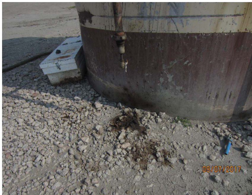
Photo #11 – Localized, oil-stained soil and gravel beneath 1” valve on SW side of AST located at workover rig.
