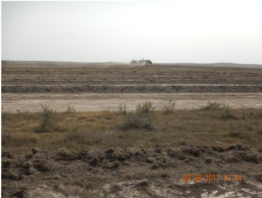
Photo 1. Photo taken from the western location, facing East. Topsoil salvage operations IN-PROCESS. Temporary BMP (i.e., ditch) installed around in the entire perimeter of the location.
