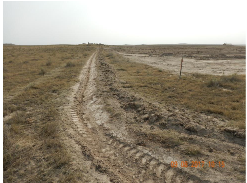
Photo 2. Photo taken from the northwest location, facing East. Topsoil salvage operations IN-PROCESS. Temporary BMP (i.e., ditch) installed around in the entire perimeter of the location.
