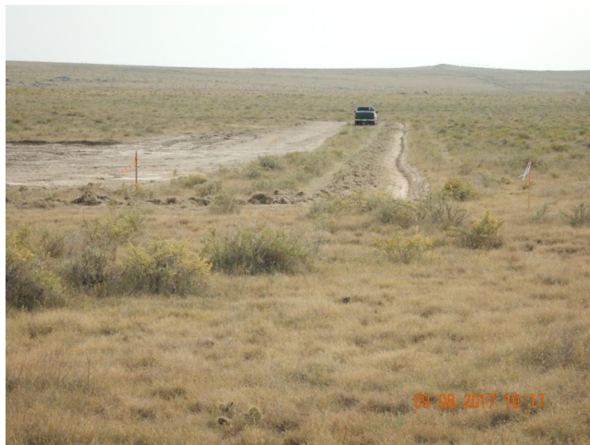
Photo 4. Photo taken from the Southwest location, facing East. Topsoil salvage operations IN-PROCESS. Temporary BMP (i.e., ditch) installed around in the entire perimeter of the location.
