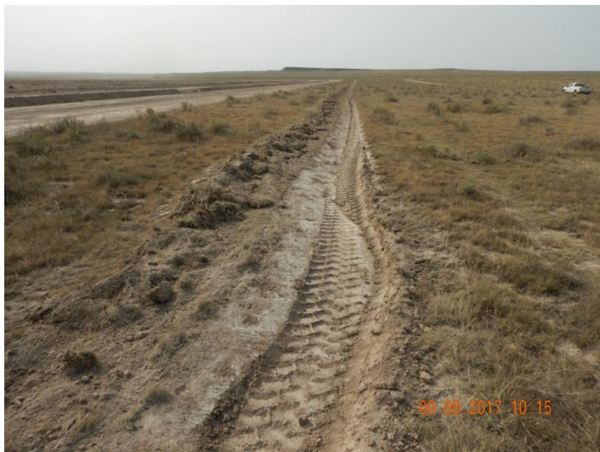
Photo 3. Photo taken from the northwest location, facing South. Topsoil salvage operations IN-PROCESS. Temporary BMP (i.e., ditch) installed around in the entire perimeter of the location.
