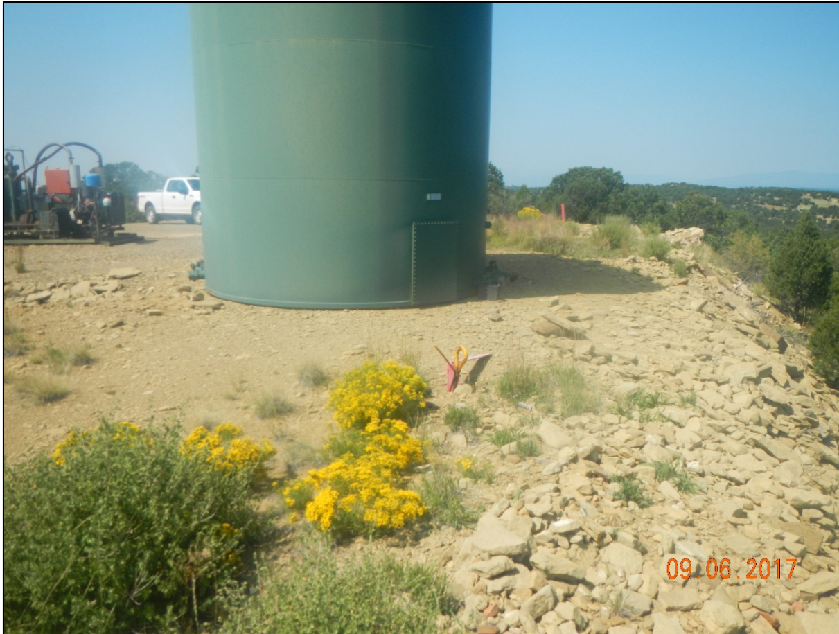
Photo 2. Facing northwest at the backside of the tank that is not in use and has no secondary containment..
