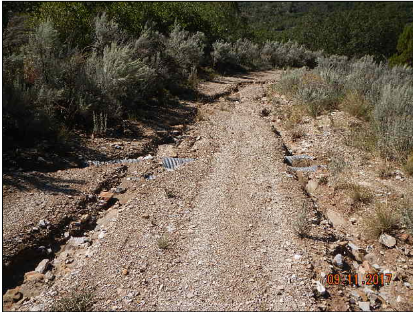
Photo 1. Access road is heavily eroded.
