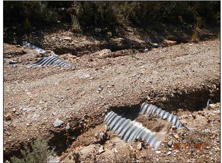
Photo 2. Culvert is damaged and non-functional.
