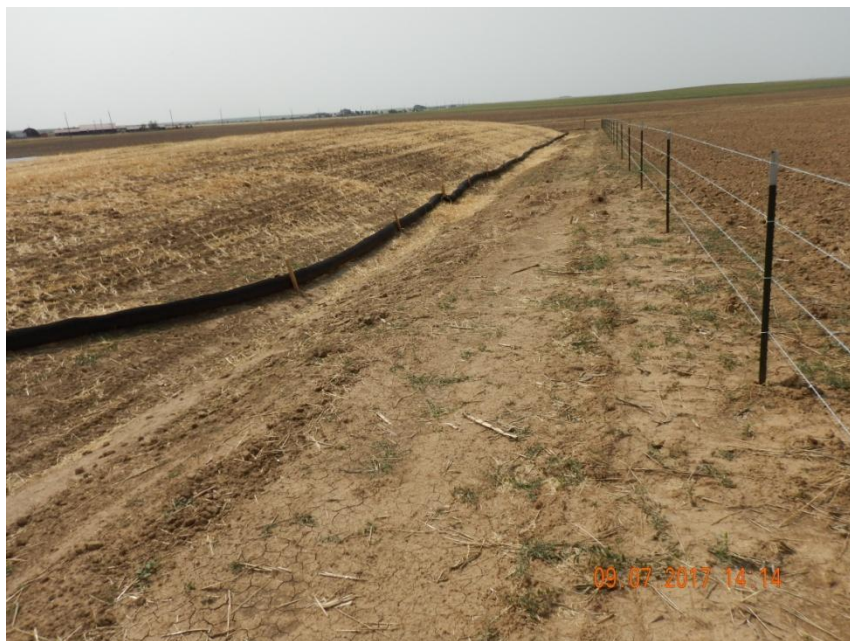
Photo 5. Photo taken from the northern location, facing West. Ditch BMP has been installed around well pad perimeter and portions of the outer perimeter.
