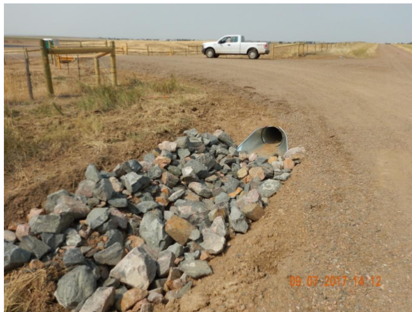
Photo 2. Photo taken from the entrance of location, facing North. A culvert installed at the entrance with a stabilized inlet and outlet area.
