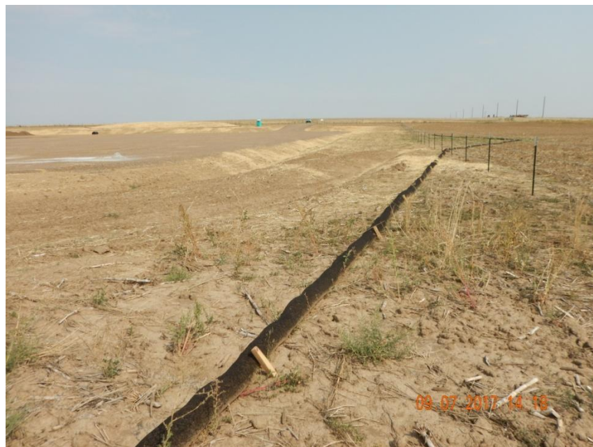
Photo 8. Photo taken from the southwest location, facing East. Ditch BMP has been installed around well pad perimeter and portions of the outer perimeter, in addition to filterxx BMP outside of the ditch BMP. A small portion along the southern perimeter outside of the fenced area was not mapped but appeared to be oil and gas disturbances. Ditch and filterxx BMP observed outside the fenced area.
