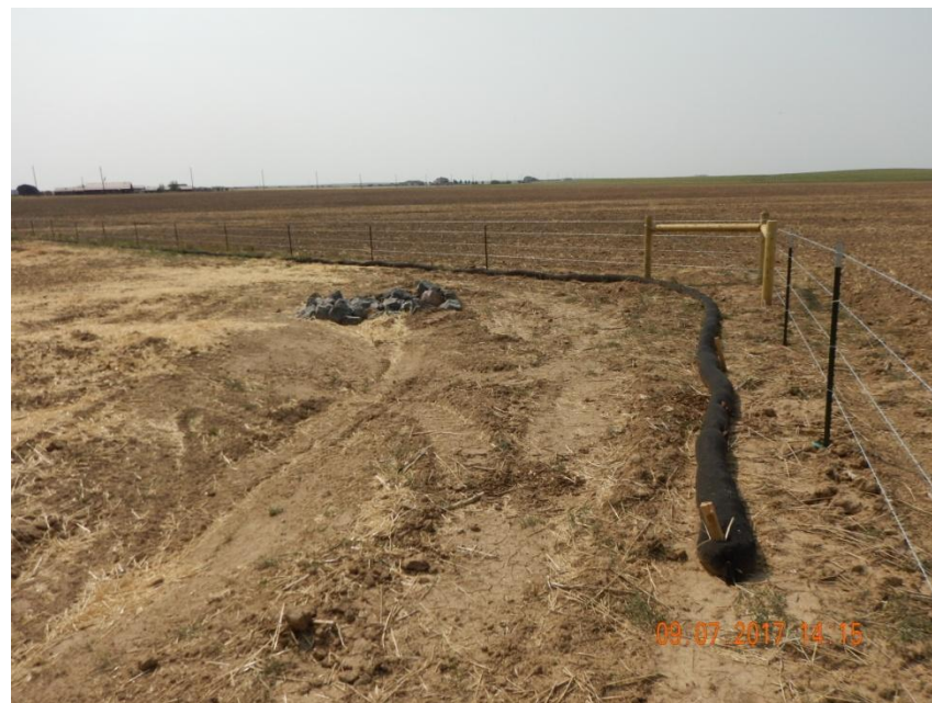
Photo 6. Photo taken from the northwest location, facing West. Ditch BMP that installed around the northern topsoil stockpile ends at a stabilized area made of rip-rap. Filtrexx BMPs have been installed along the northwestern, western, and southern location perimeters.
