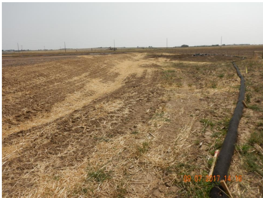
Photo 7. Photo taken from the northwest location, facing South. Ditch BMP installed around the well pad perimeter is directed to the western sediment trap- see photo 9.
