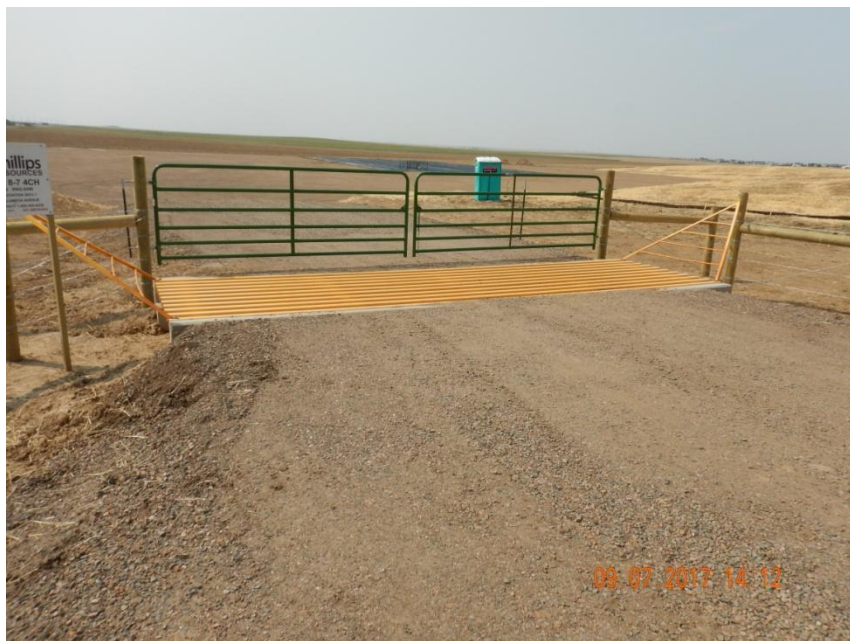
Photo 3. Photo taken from the entrance of location, facing West. Cattle guard installed at the entrance of location.
