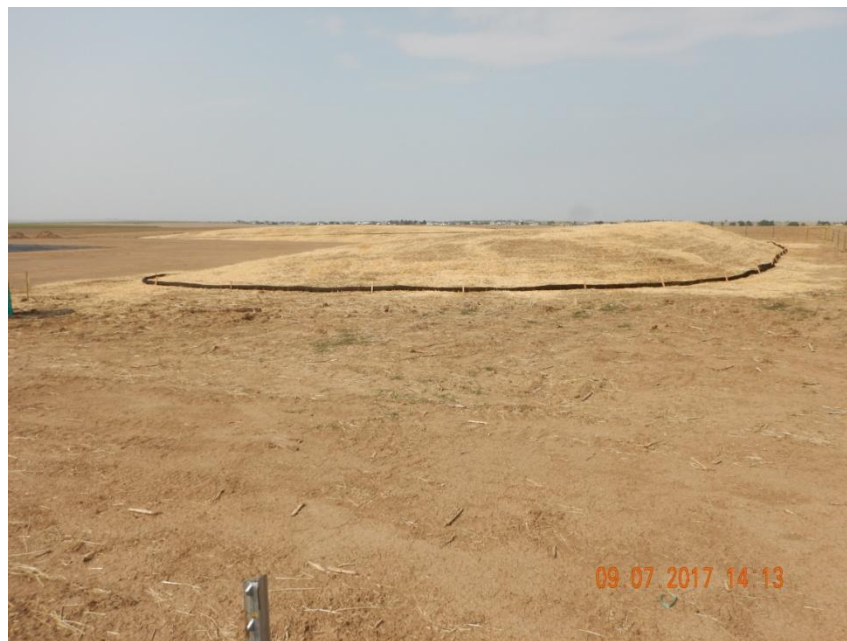
Photo 4. Photo taken from the eastern location, facing North. Appears topsoil has been salvaged and stored along the eastern and northern well pad perimeters. Topsoil has been mulched with a filtrex wattle installed around the toe of slope.
