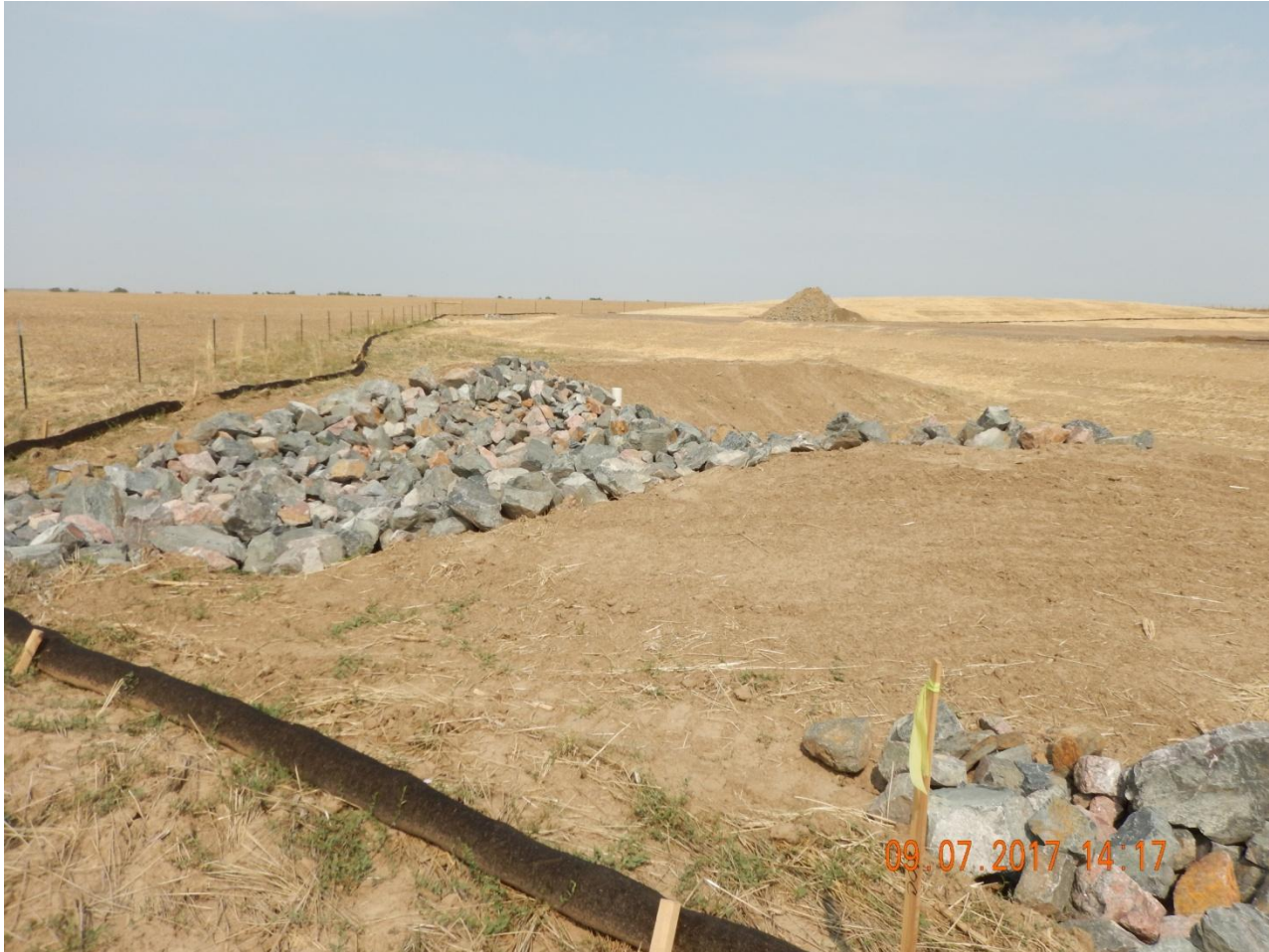
Photo 9. Photo taken from the western sediment trap, facing North. Sediment trap has been installed with a stabilized outlet, in addition to filtrex BMP along the outer perimeter.
