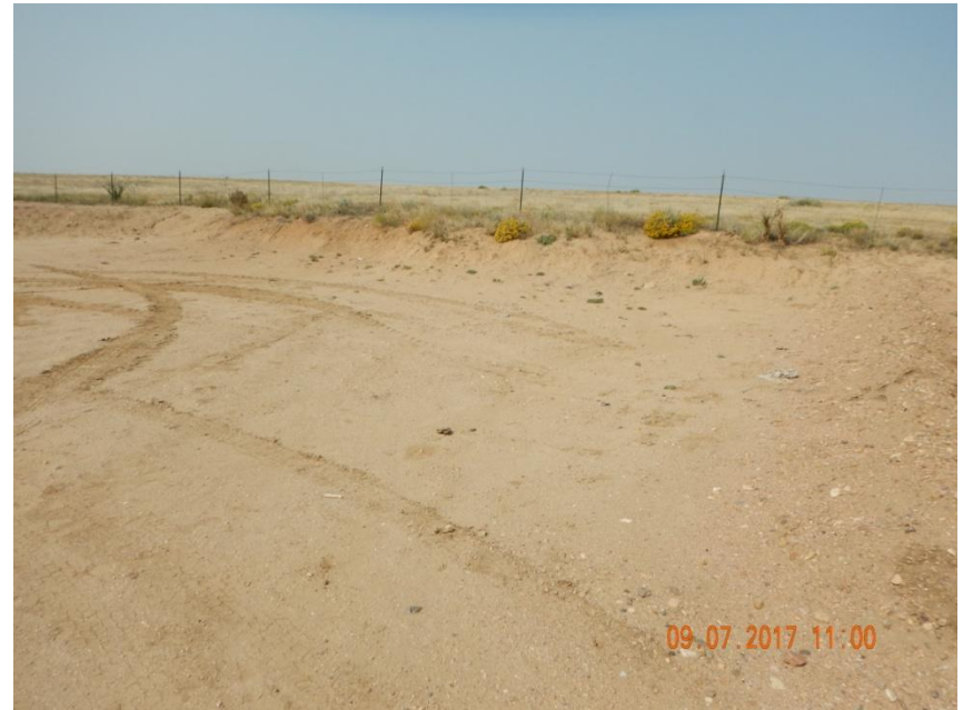
Photo 4. Photo taken September 7, 2017 from the previous photo location, facing Southwest. Does not appear the Operator has made repairs to the rill erosion along the cut slope. Does not appear the Operator has installed a BMP to prevent erosion and stabilize the production area.
