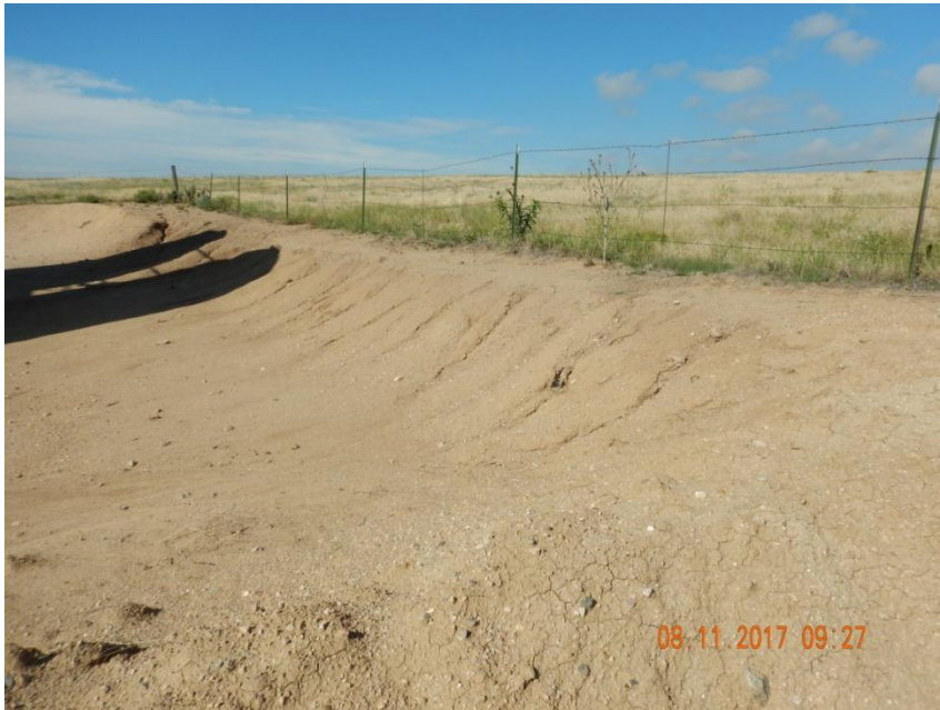
Photo 3. Photo taken August 11, 2017 from the western location, facing Southwest. Rill erosion occurring throughout the cut slope contributing to sediment discharge off location. Cut slope needs to be stabilized to prevent erosion and stabilize the production area.
