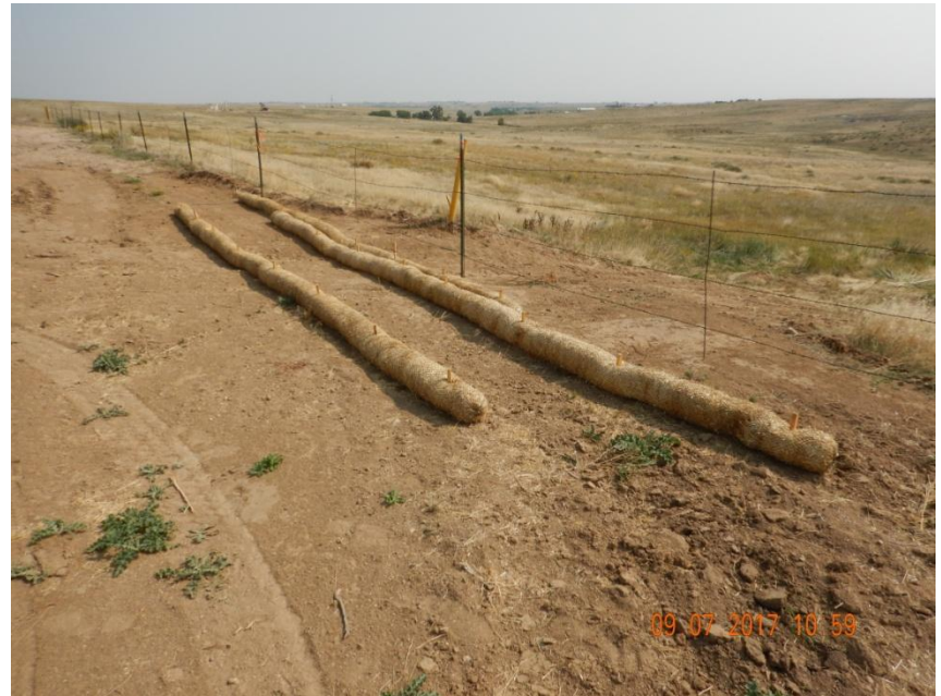
Photo 2. Photo taken September 7, 2017 from the previous photo location, facing Northeast. Appears to Operator has repaired the erosion. Operator has installed wattle BMPs but BMP has not been properly installed.
