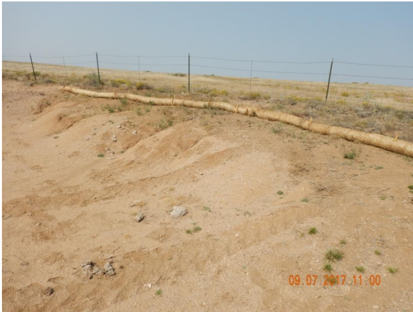
Photo 5. Photo taken September 7, 2017 from the northwestern location, facing Southwest. Does not appear the Operator has made repairs to the rill erosion along the cut slope. Operator has installed wattle BMPs but BMP has not been properly installed.
