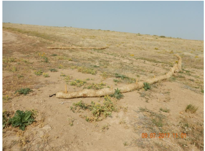
Photo 6. Photo taken from the second discharge point off the main access road, facing North. Operator has installed wattle BMPs but BMP has not been properly installed.
