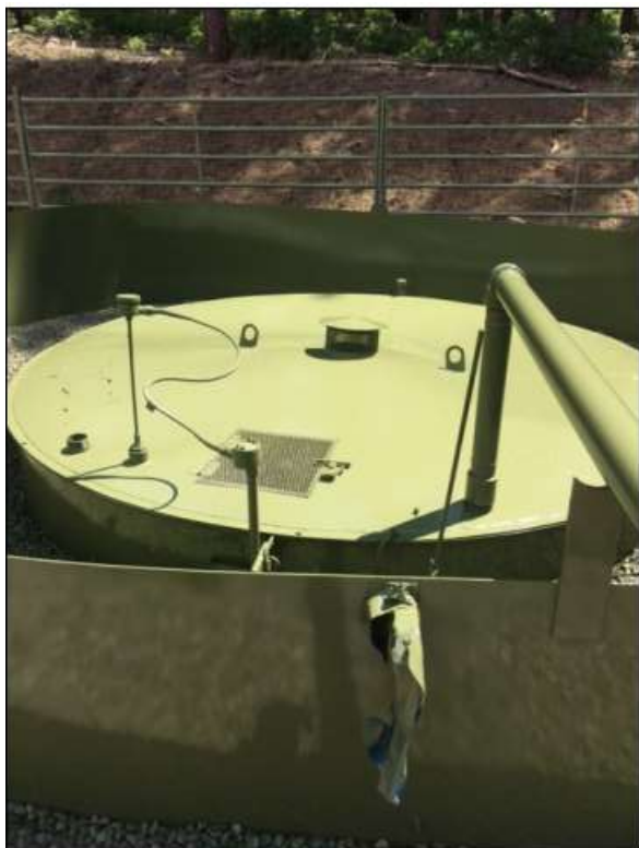
Tank and tank metal containment ring painted
