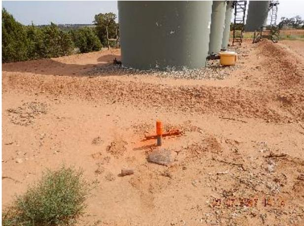
**Photo 11: Unused risers outside produced water tank berms.**
