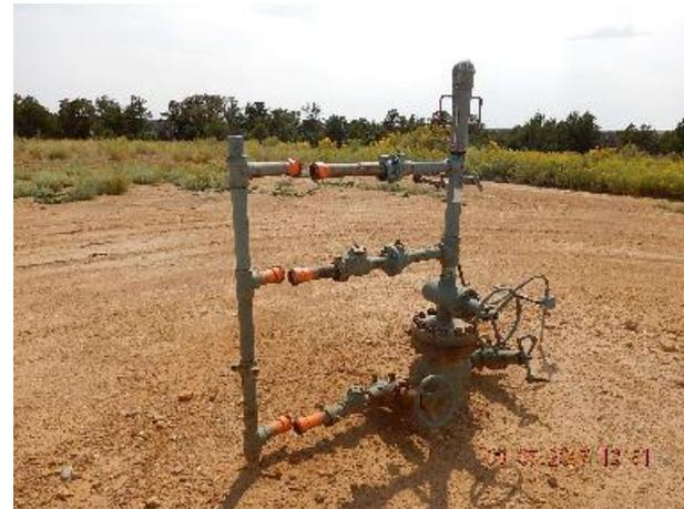
Photo 2: Disconnected wellhead and riser.
