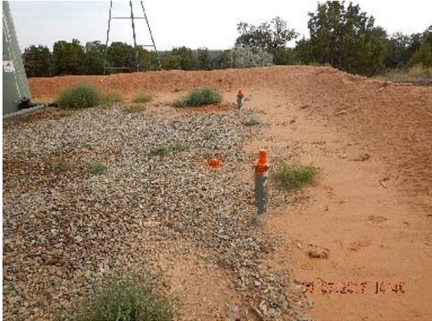
**Photo 13: Unused risers inside oil tank battery. Impacted soil and gravel in left of frame.**
