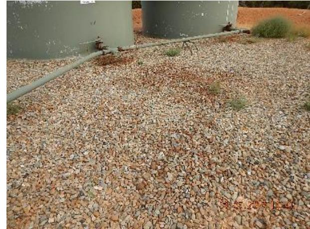
**Photo 14: Impacted soil and gravel under valves and out from tank.**
