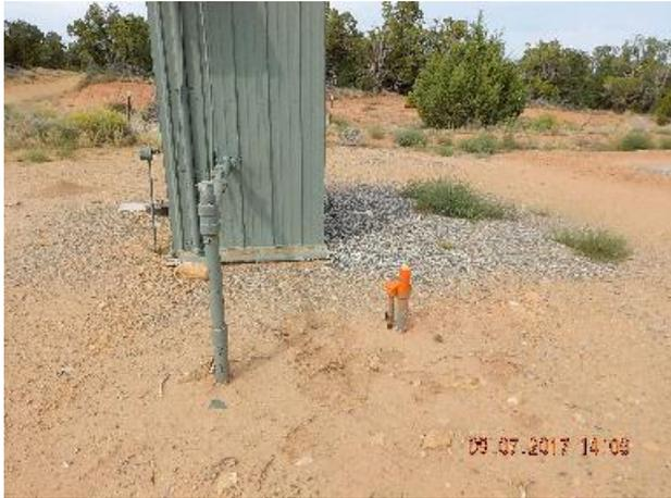
**Photo 9: Unused risers at gas meter shed.**
