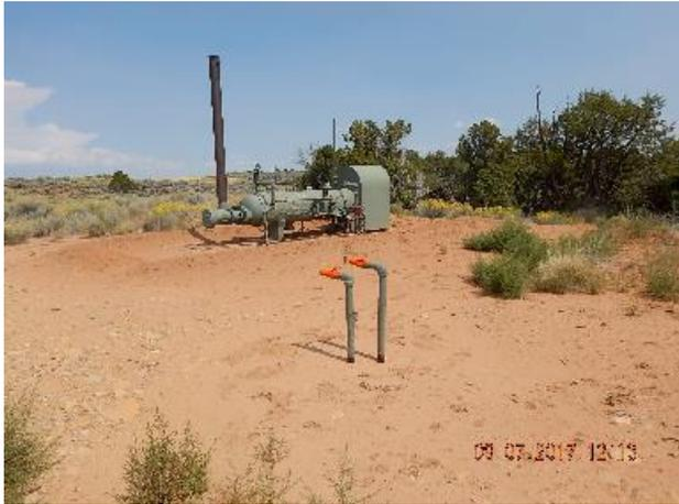
**Photo 7: Unused riser S side of separator.**
