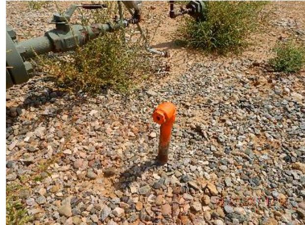
**Photo 6: Unused riser at wellhead.**
