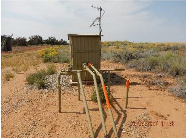
**Photo 5: Unused riser and abandoned flowline at meter run.**
