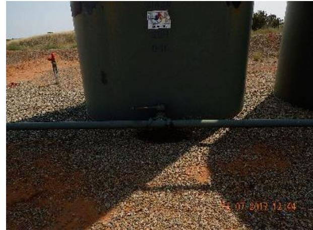
**Photo 14: Impacted soil and gravel under valve. One of several that need to be cleaned up.**
